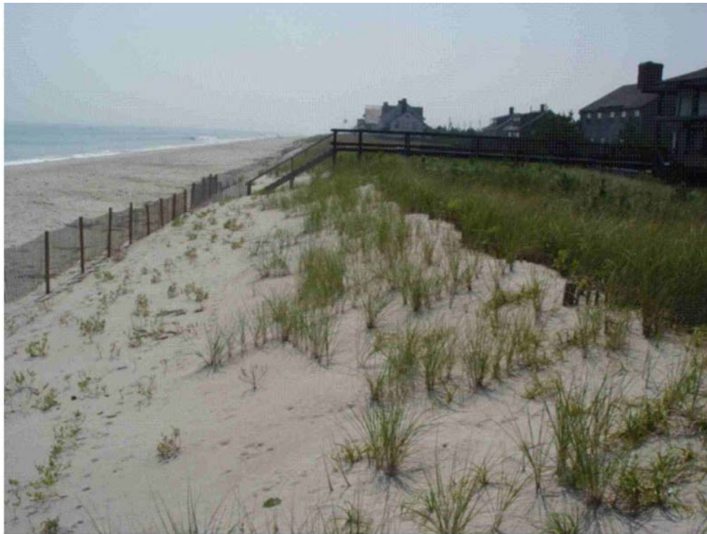
Photoplate 3a. Photo taken September 13, 2005 in Mantoloking, NJ. The sparsely vegetated seaward slope of the dune is due to a bulldozing effort in 2003 following several small northeast storms that cut to the edge of the dense grass leaving a 6 to 8-foot scarp in the dunes. Note the dune cross over to the south.
