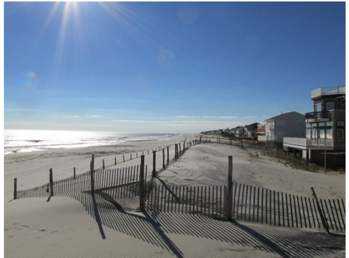
The Webster Avenue photos were taken from the crest of the restored dune (left taken October 31, 2014 and right taken December 15, 2015). The dune was restored to its original position and elevation in 2013 and has remained consistent throughout 2014-2015.
