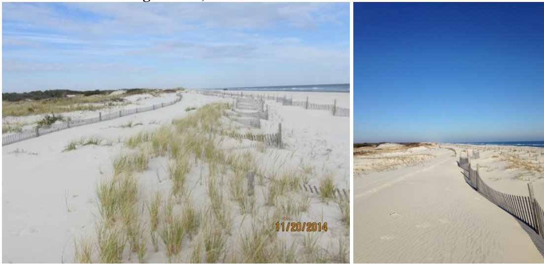
The photos (left November 20, 2014 and right December 7, 2015) that were taken at this Island Beach State Park location show the condition of the dune via sand fencing and natural recovery. The dunes here are lower than at the other two sites within the park, but the dune field is nearly 200 feet wide.
