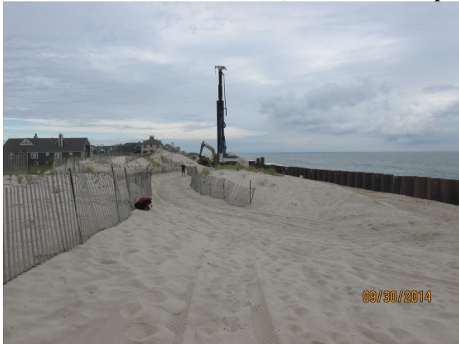
On the left (taken September 30, 2014) shows the installation of the southern section of the steel bulkhead. The right photo (December 14, 2015) is the view from the top of the new dune that covers the bulkhead. Sand was brought in from a non-beach source for the construction.
