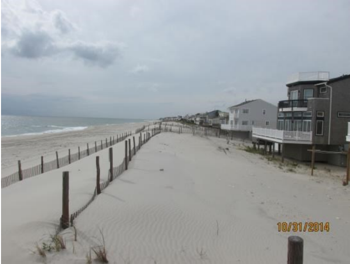
The Webster Avenue photos were taken from the crest of the restored dune (left taken October 31, 2014 and right taken December 15, 2015). The dune was restored to its original position and elevation in 2013 and has remained consistent throughout 2014-2015.
