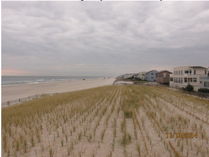
The photos (left taken November 13, 2014 and right taken September 16, 2015) show the nearly unchanged condition of the engineered dune at Tranquility Drive. This site was included in the emergency federal beach nourishment project that was completed in spring 2013.
