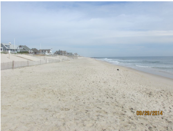
Both photos (left taken September 29, 2014 and right taken December 14, 2015) show the condition of the berm at the Bay Head location. While the berm appears wider in the photos, the profile lost volume (-20.31 yd 3 /ft.) during this time period, predominantly below the 0.0 ft. datum.
