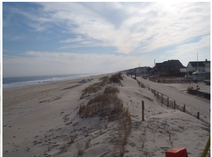
At the Lavallette site, the photos (left taken September 30, 2014) and right (taken December 11, 2015) show the condition of the dune that was created by pushing sand against the boardwalk following Hurricane Sandy. Some sand accumulated at the seaward base of the dune after the June 2015 survey.
