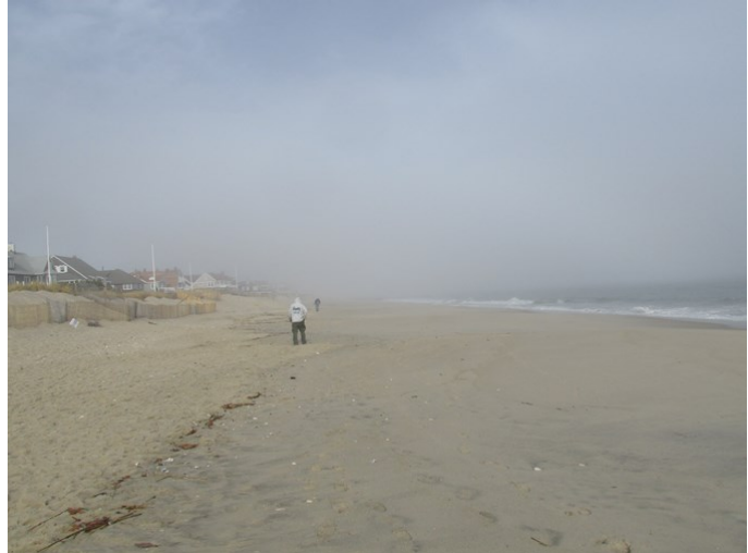
Both photos (left taken September 29, 2014 and right taken December 14, 2015) show the condition of the berm at the Bay Head location. While the berm appears wider in the photos, the profile lost volume (-20.31 yd 3 /ft.) during this time period, predominantly below the 0.0 ft. datum.
