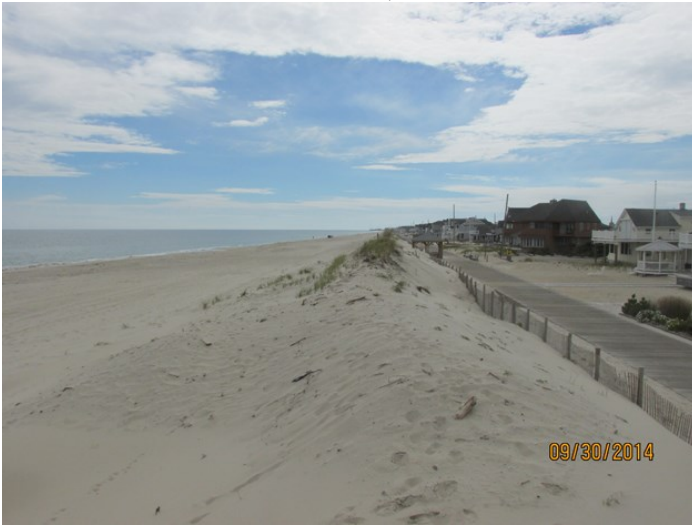
At the Lavallette site, the photos (left taken September 30, 2014) and right (taken December 11, 2015) show the condition of the dune that was created by pushing sand against the boardwalk following Hurricane Sandy. Some sand accumulated at the seaward base of the dune after the June 2015 survey.
