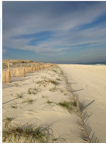
The photo on the left (taken November 14, 2014) shows the beach has remained constant from its 2013 state with some minor growth in the dune. The right photo (taken December 7, 2015) shows sand accumulating on the landward side of the seaward-most dune fence.
