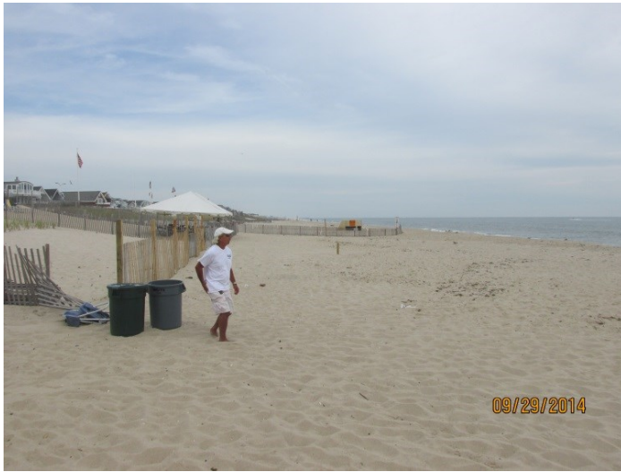
The Maryland Avenue profile is located south of Manasquan Inlet. The photos (left taken September 29, 2014 and right taken December 14, 2015) show a maintained beach. Installation of sand fencing seaward of existing fence is a local effort to capture wind-blown sand. Volume changes across the profile were minimal (0.72 yd 3 /ft.) between fall 2014 and fall 2015.
