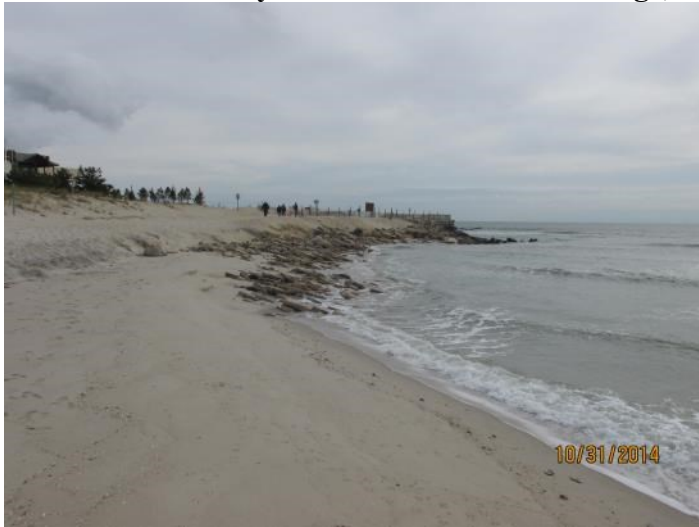
The Holgate Unit photos (left taken October 31, 2014 and right taken December 15, 2015) show the changing conditions of the berm and surf zone. This site is immediately south of the Long Beach Island terminal groin which influences the amount of sand that is available to this downdrift beach. The profile was completely overwashed during Hurricane Sandy.
