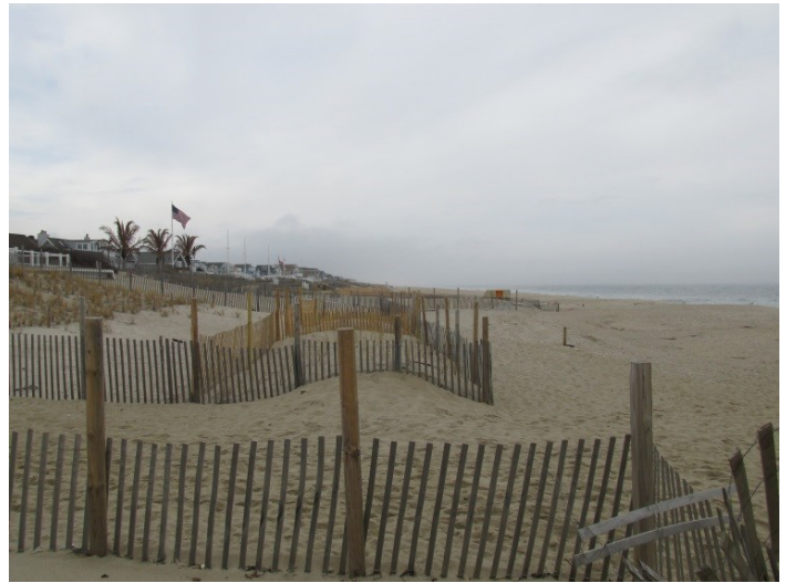
The Maryland Avenue profile is located south of Manasquan Inlet. The photos (left taken September 29, 2014 and right taken December 14, 2015) show a maintained beach. Installation of sand fencing seaward of existing fence is a local effort to capture wind-blown sand. Volume changes across the profile were minimal (0.72 yd 3 /ft.) between fall 2014 and fall 2015.
