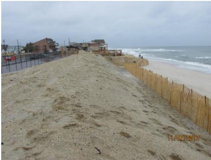
On the left, (taken November 7, 2013) the restored boardwalk was moved landward of its original position (about 25 feet) with a new dune composed of recovered sand. A year later (right) the dune has not been planted or further augmented, but the beach is a little wider.
