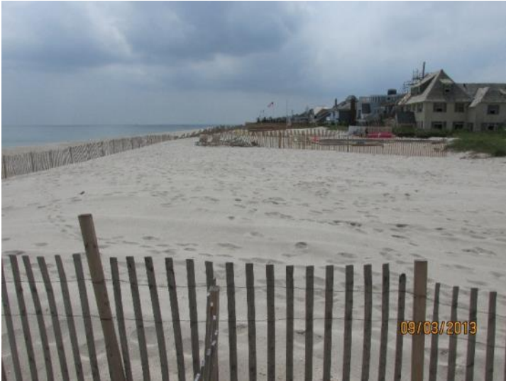
On the left, (September 3, 2013) sand recovered from the overwash deposits inland was returned to the beach to cover the rocks and raise the dune elevation. By September 29, 2014 the grass was planted and dune toe fencing was in place.
