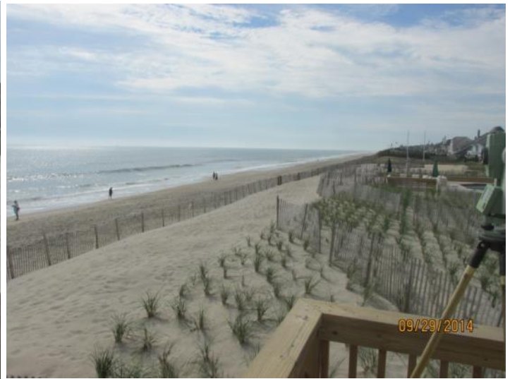
On the left, (September 3, 2013) sand recovered from the overwash deposits inland was returned to the beach to cover the rocks and raise the dune elevation. By September 29, 2014 the grass was planted and dune toe fencing was in place.
