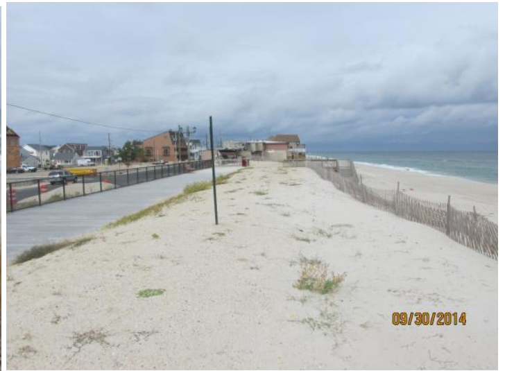
On the left, (taken November 7, 2013) the restored boardwalk was moved landward of its original position (about 25 feet) with a new dune composed of recovered sand. A year later (right) the dune has not been planted or further augmented, but the beach is a little wider.
