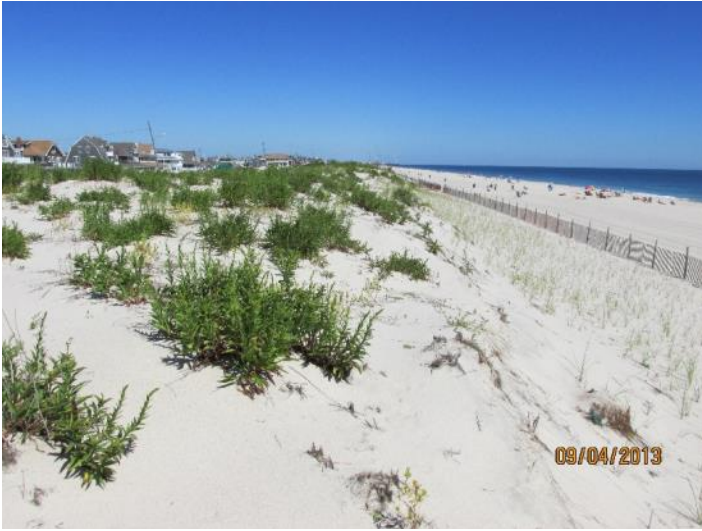
The photo on the left (taken September 4, 2013) shows the results of local efforts to restore the eroded dune and trap sand at a new dune fence system. In the subsequent year, the beach has remained constant with some minor growth in the dune.
