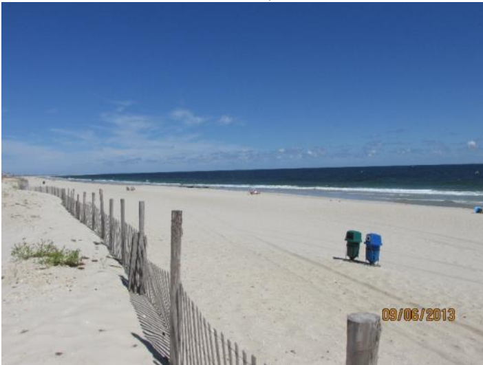
The right photograph was taken Sept. 6, 2013. A year later, the fencing appears to have accumulated some sand at the crest and developed a berm with more sand offshore in a bar.
