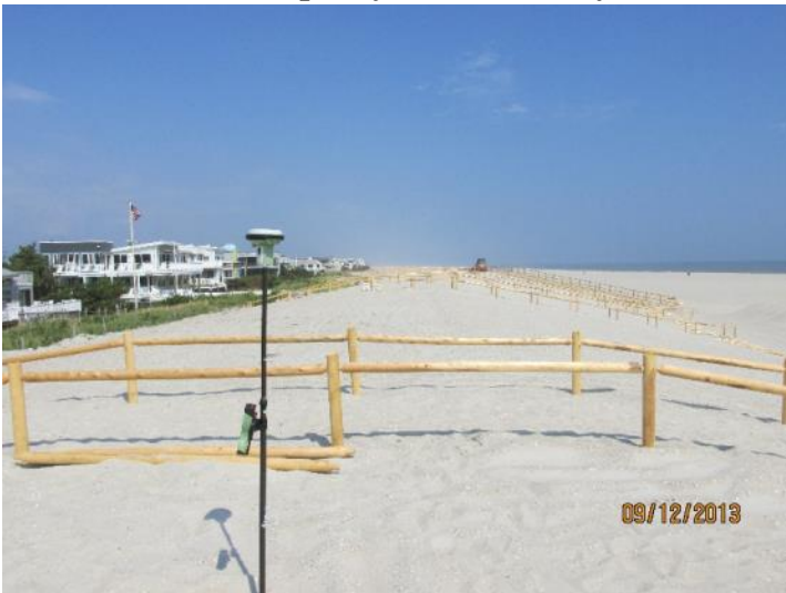
The Tranquility Drive site was included in the 2010 USACE beach nourishment project. The photo on the left (taken on September 12, 2013 – a year post-Sandy) shows the results of ACOE efforts in restoring the dune and berm to design template specifications. A year later (November 13, 2014) grass was in place and sand was accumulating at the dune toe.
