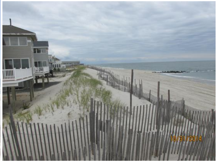
The photographs above were taken on September 24, 2013 (left) and October 31, 2014 (right). Both images show the view of Dolphin Avenue (site 136) looking north. The lost dune was replaced by a smaller feature using sand hauled back to the beach from inland deposits. Growth since fall 2013 was confined to the lower seaward dune slope and offshore.
