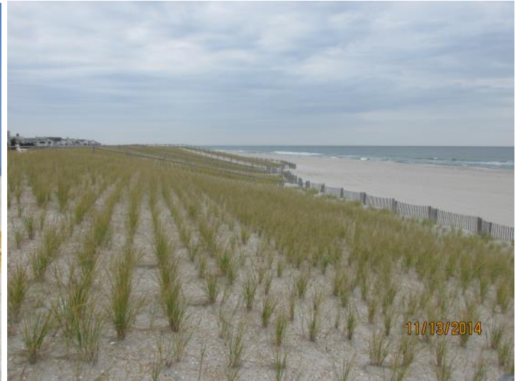
The Tranquility Drive site was included in the 2010 USACE beach nourishment project. The photo on the left (taken on September 12, 2013 – a year post-Sandy) shows the results of ACOE efforts in restoring the dune and berm to design template specifications. A year later (November 13, 2014) grass was in place and sand was accumulating at the dune toe.
