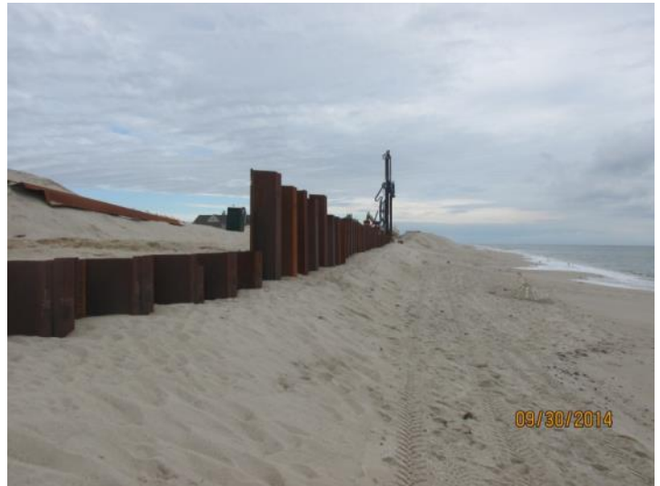
On the left (taken September 5, 2013) shows a restored dune cross section combined with a berm deposited over the summer of 2013. The fall view from September 30, 2014 shows work in progress installing the steel sheets making up the bulkhead extending south into Brick Township from near the Bay Head boundary in Mantoloking.
