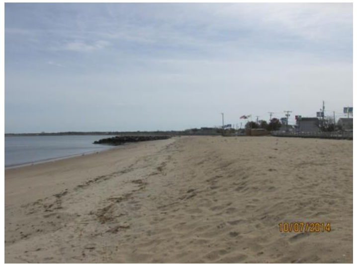
This site was moved to the public bathing beach in 2009. The photograph on the left shows the shoreline on October 7, 2013 following the addition of 14,000 cu. yds. of added sand. The photo on the right shows the adjustment in beach width over a year following the municipality’s efforts in replacing lost sand following Sandy (taken on October 7, 2014).
