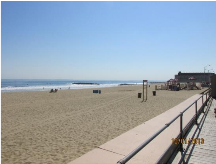
This site is the northernmost site included in the Federal shore protection southern project segment. The left photo (taken on October 1, 2013) showed natural sand recovery. Natural recovery permitted 17.79 yds 3 /ft. in offshore deposition to return to the beach. The federal project added 92.68 yds 3 /ft. and produced a 100-foot shoreline advance.
