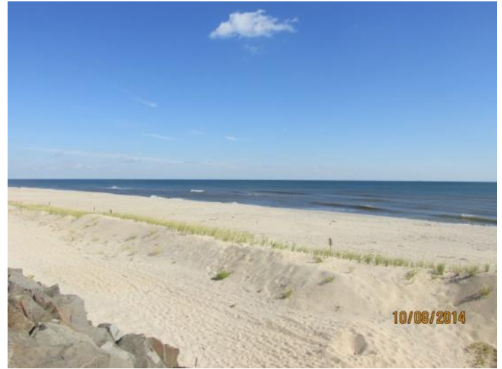
This site is near the northern limit of the initial Federal shore protection. The left side shows the results of the placement of 40.12 yds 3 /ft. of new sand on the beach by Oct 17, 2013, while the right side (Oct. 8, 2014) shows the added dune.
