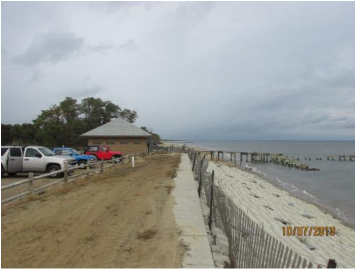
This site was enhanced by adding slope protection to the eroding uplands bluff prior to Sandy. The photograph on the left shows the shoreline on October 7, 2013. The right picture was taken October 7, 2014 as a massive beach restoration was being completed.
