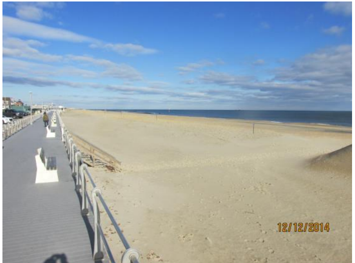
Boardwalk damage was restored and 39.16 yds 3 /ft. in lost sand returned by Sept 26, 2013 from deposits formed offshore. Modest additions were made by the ACOE during 2014 (23.81 yds 3 /ft.) and the beach was wider.
