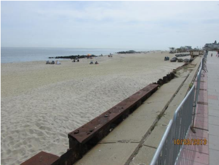
Natural recovery from the offshore deposits added 22.72 yds 3 /ft. to the beach prior to 2014 ACOE restoration activities. The right photograph taken November 18, 2014 shows a wider beach relative to the rock groins compared to the left photo.
