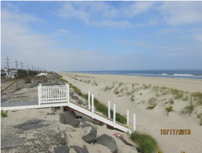
The left view shows ACOE pumped sand back to the original design cross section and the sand the storm pushed up the seaward face of the seawall was extracted and formed into the dune seen on the left view October 17, 2013. A wide, new berm accumulated between February and October 2014 adding 42.25 yds 3 /ft. to the profile.
