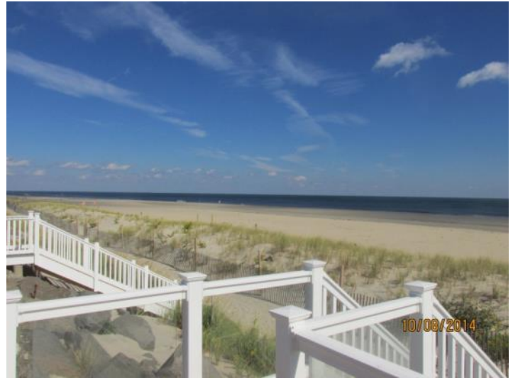
The left view shows ACOE pumped sand back to the original design cross section and the sand the storm pushed up the seaward face of the seawall was extracted and formed into the dune seen on the left view October 17, 2013. A wide, new berm accumulated between February and October 2014 adding 42.25 yds 3 /ft. to the profile.
