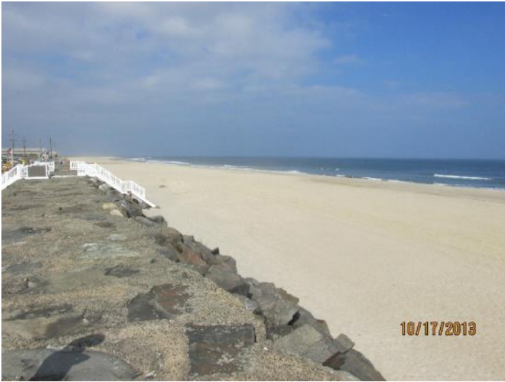
This site is near the northern limit of the initial Federal shore protection. The left side shows the results of the placement of 40.12 yds 3 /ft. of new sand on the beach by Oct 17, 2013, while the right side (Oct. 8, 2014) shows the added dune.
