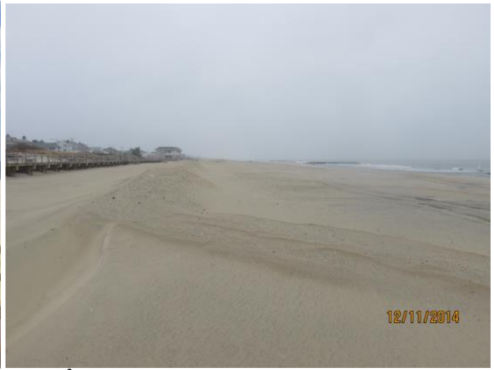
A massive effort restored the boardwalk by Sept 26, 2013 and 31.40 yds 3 /ft. in eroded beach/dune sand returned to the beach naturally. By December 11, 2014 (right) the ACOE had added 40.47 yds 3 /ft. in new sand advancing the shoreline by 13 feet.
