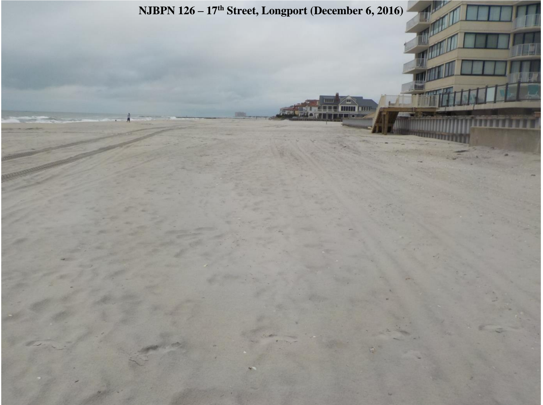
Figure 444. NJBPN site 126 is located at 17 th Street in Longport. The view here is looking south along the Longport beach toward the terminal rock groin at 11 th Street. There is approximately 150 ft of dry recreational beach seaward of the seawall/revetment, no attempt has been made to establish a dune feature in this region.
