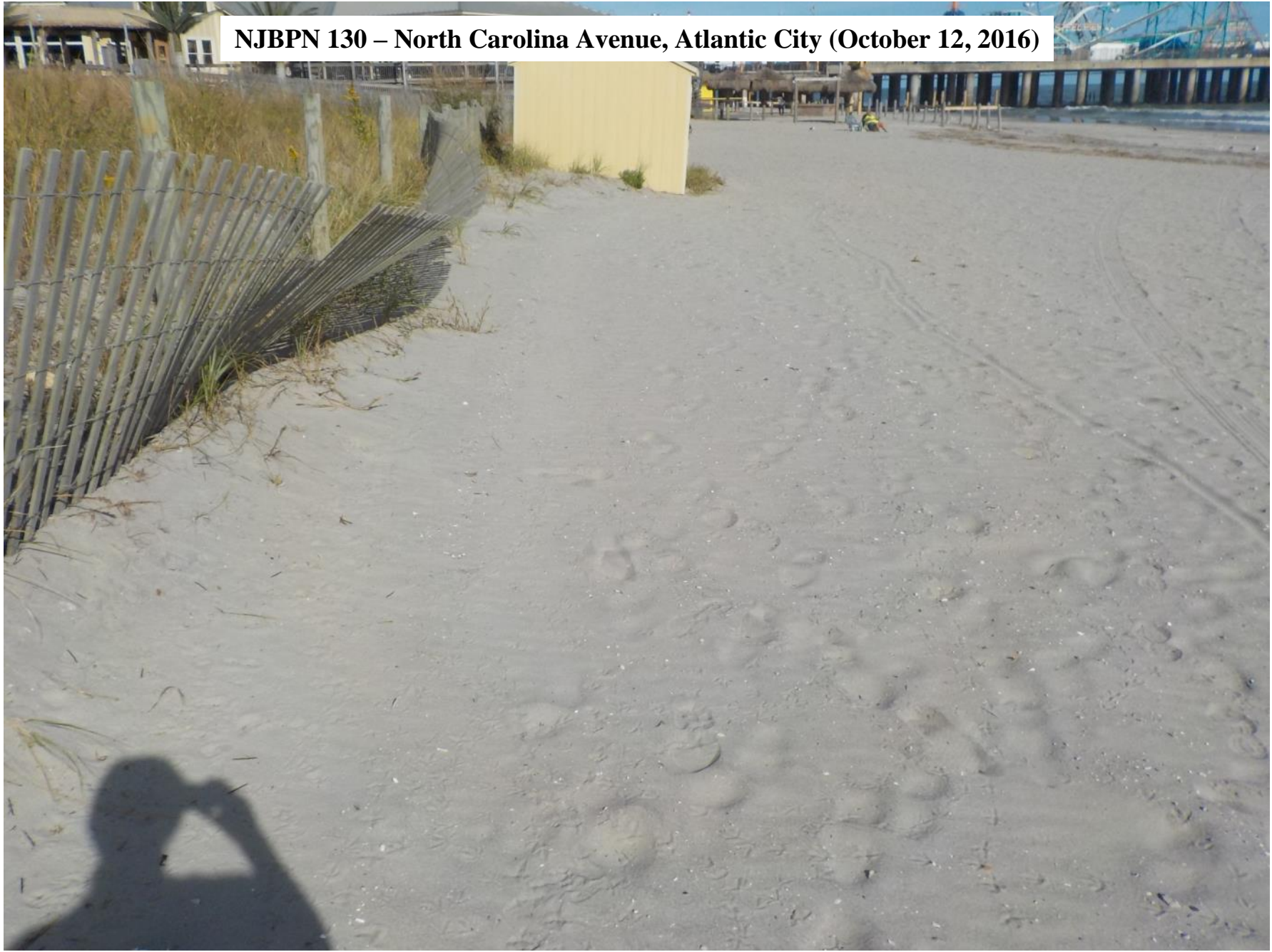
Figure 420. NJBPN site 130 is located at North Carolina Avenue in Atlantic City. View is along the seaward dune toe to the north with the Steel Pier in the background. The beach has eroded but still remains wide enough to support the dune in its current location and configuration.
