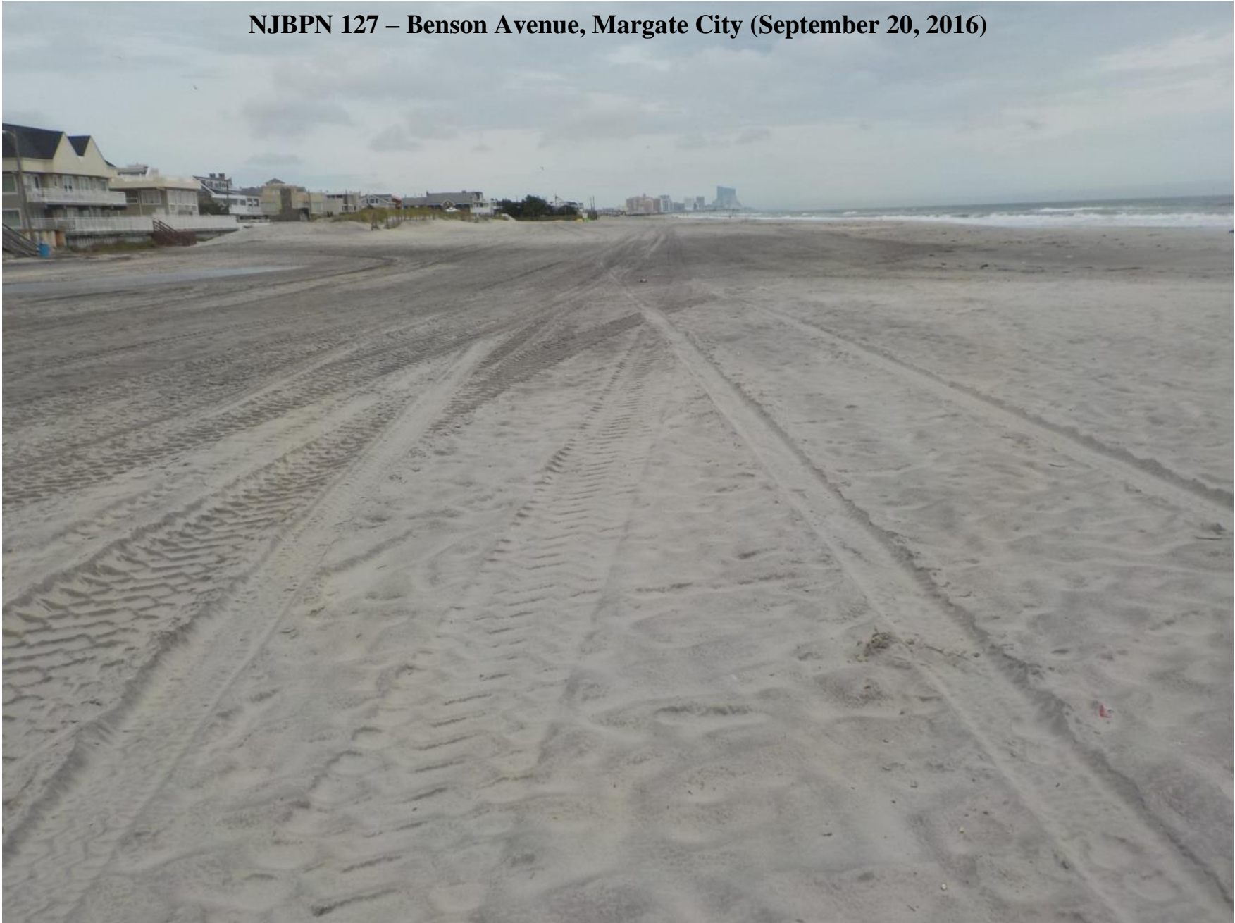
Figure 438. NJBPN site 127 is located at Benson Avenue in Margate City. View here is looking north along the Margate City beach. There is approximately 350 ft of dry recreational beach width seaward of the street end bulkhead/revetment but with no dune development along this profile transect.
