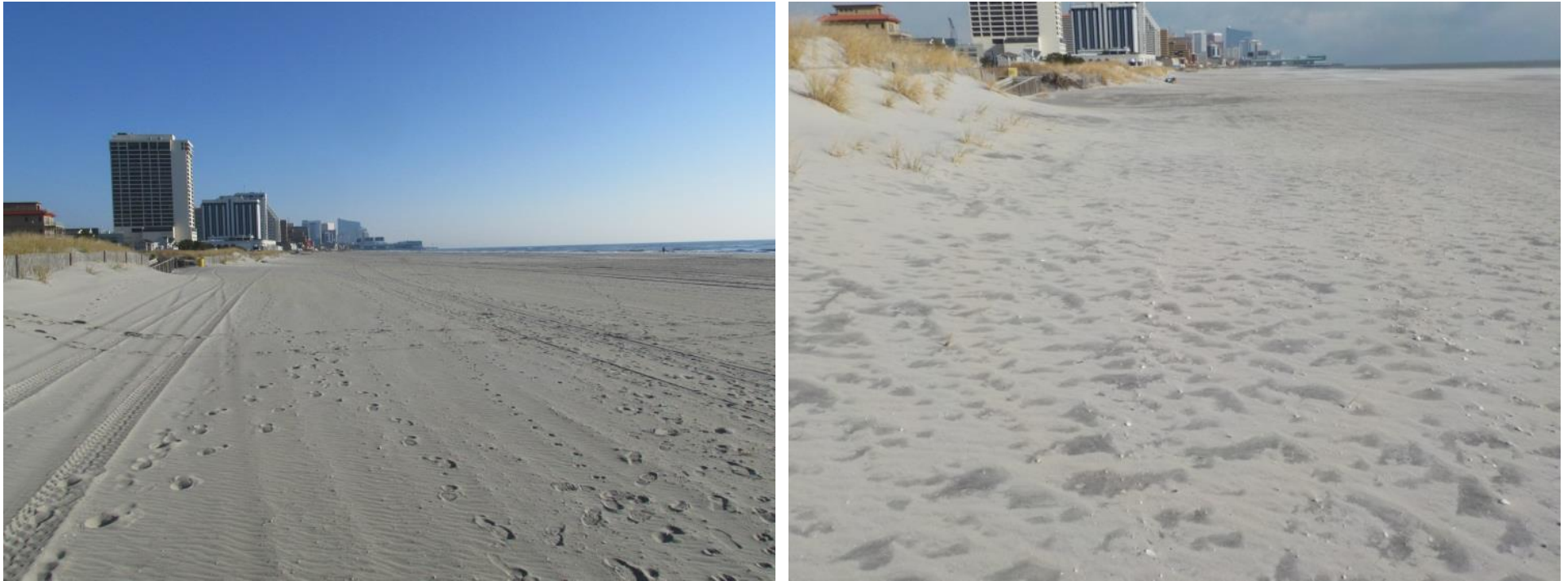
Figure 427a & 427b. Raleigh Avenue is located near the middle of the federal shore protection project on Absecon Island, the dune and beaches are relatively stable. The photo on the left (December 10, 2015) is taken looking north along the well-developed seaward dune toe. The photo on the right was taken December 15, 2016 and shows sand accumulated along the seaward dune fence.
