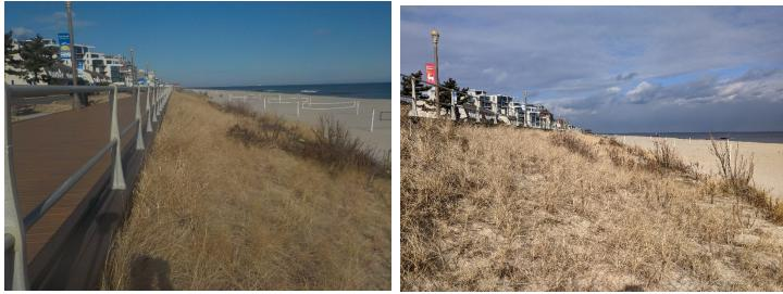
The bluff revetment is the first element in the survey with a 230-foot wide beach to the berm (Jan. 6, 2020 on left). No dune exists at the foot of the revetment, but the beach width remained relatively constant (January 20, 2021 on right).
