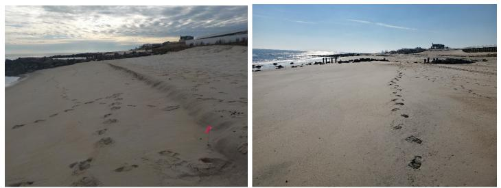
This site is located on the highest point along the bluff shoreline. By January 7, 2020 erosion had fully exposed the rock groin and pushed the beach berm nearly to the main shore-parallel bulkhead. The right view taken January 12, 2021 shows a much less exposed groin following maintenance nourishment.
