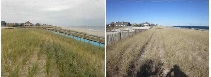
The beachfill was completed at the Brick Township Public Beach #3 profile site in summer 2018 with the engineered dune covering the steel bulkhead. The photos show the condition of the dune (left taken November 5, 2019 and right taken November 18, 2020). The dune remained in position and elevation throughout 2020.
