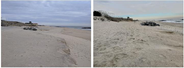
This site fronts a private home at the bluff. As of Jan. 7, 2020, the beach developed a scarp near the rock revetment with sand deposited as a repair berm seaward of the scarp on the left side view. The January 8, 2021 view presents a very similar perspective with the rock revetment having increased exposure.
