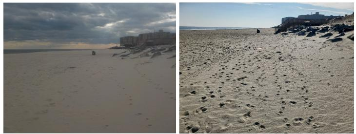
This site was the southern location within Phase I of the federal project. On the left, the rock wall was partially buried in wind-transported sand (Jan 16, 2020). The right-hand view on Jan. 12, 2021 shows the rock toe of the revetment further buried in wind-deposited sand.
