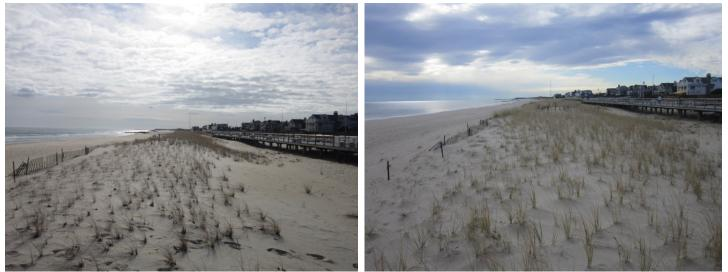
The photo on the left (Jan 10, 2020) shows the grass was partially buried by added wind deposition and the damaged fence was still unrepaired. The December 7, 2020 view on the right shows the fence once again, unrepaired but still capturing a minor amount of sand.
