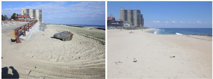
As of January 6, 2020, the rock wall was complete, and the sand pipeline was in place on the beach. The right photo, taken January 13, 2021, shows the beach with the offset in the shoreline produced by the groin at the property line.
