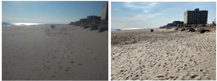
The left view is from Jan. 6, 2020 and shows the sand ramped up against the rock revetment protecting the beach bluff. The right view from Jan. 13, 2021 shows that grass did develop between rocks in that wind deposited sand.
