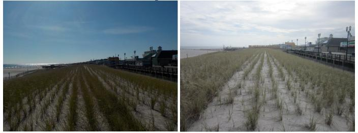
At the Franklin Avenue profile, an engineered dune was constructed within the federal beachfill in January 2019. No dune existed prior to the beachfill. The dune remained stable through 2020 (left photo taken November 6, 2019 and right photo taken November 11, 2020).
