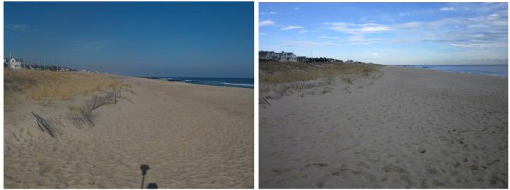
The Nov. 25, 2019 view (left photo) is at the toe of the dunes showing minor scarping and fence damage, like that seen to the north at site 15801. The right-hand side photo shows the damaged fence further buried, with dune grass growth proceeding seaward beyond the fencing.
