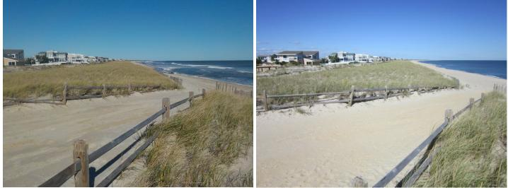
The photos show the vegetated engineered dune that was constructed at La Baia Street in 2016 (left photo taken November 1, 2019 and right photo taken October 8, 2020). The dune and berm remained in relative position and elevation in 2019-2020. Some sand accumulated along the landward side of the shore-parallel fencing that protects the dunes from foot traffic.
