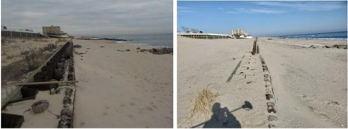
Located in the Elberon groin field, this location was completed during 2016 and suffered retreat, producing exposed rocks by Jan. 7, 2020. The beach was lower in elevation with the old timber bulkhead clearly visible on upper beach. The right photo, taken January 12, 2021 exhibits the beach where the groin is much less exposed, as well as sand recovering the bulkhead.
