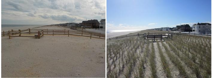
The left photo (taken November 5, 2019) shows the engineered dune which was created from the integration of sand recovered from Hurricane Sandy and the beachfill that was completed at this location in April 2019. The right photo (taken November 18, 2020) shows planted vegetation on the engineered dune.
