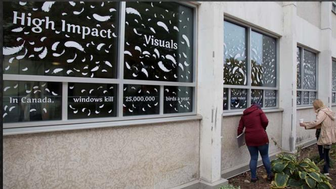
Perforated film applied to the outside of the windows eliminates reflections.
