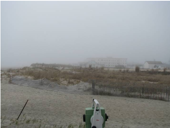
Low, wide dunes established naturally following the initial Federal beach nourishment project. Sand volumes have been relatively stable since that time (left photo taken March 22, 2012). Sandy’s storm surge and waves relocated sand from the dune and berm to both landward to the rocks and over the rocks, and to the nearshore (right photo November 21, 2012).
