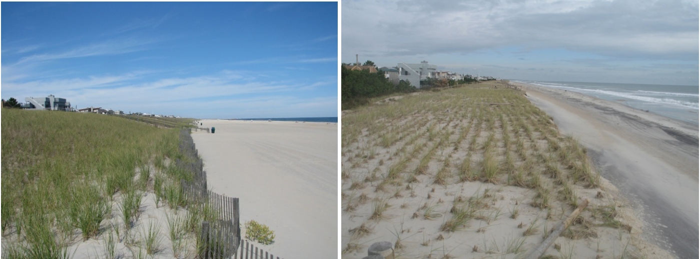
The photo on the left was taken on September 11, 2012 while the photo on the right was taken on November 2, 2012 from a similar location looking north. This site had received sand as part of the 2010 USACE beach nourishment project for Long Beach Island. The project provided ample dune and beach width enhancement and storm protection for the oceanfront properties. The post-Sandy photo shows the impact of the storm with a significant dune scarp at the seaward crest and a narrow, lower-elevation beach remaining. However there was no evidence that sand overwashed the dune at this location.
