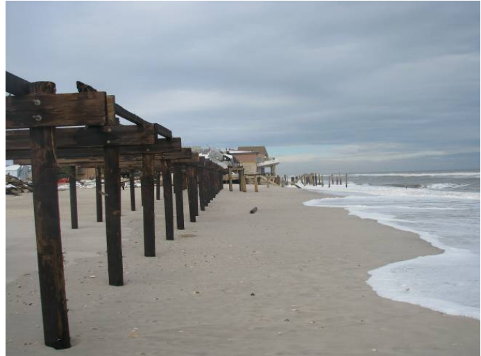
The photograph on the left (September 14, 2012) shows a modest berm and the municipal dune present prior to the storm. On the right (November 8, 2012), 68.7 yds 3 /ft of berm and dune were removed during the storm. Over 10 feet of dune height was pushed landward in overwash deposits. The boardwalk was located landward of the dunes (left) Ocean Avenue was destroyed as well as several homes. The photo on the right shows a classic flat beach created by the large waves.
