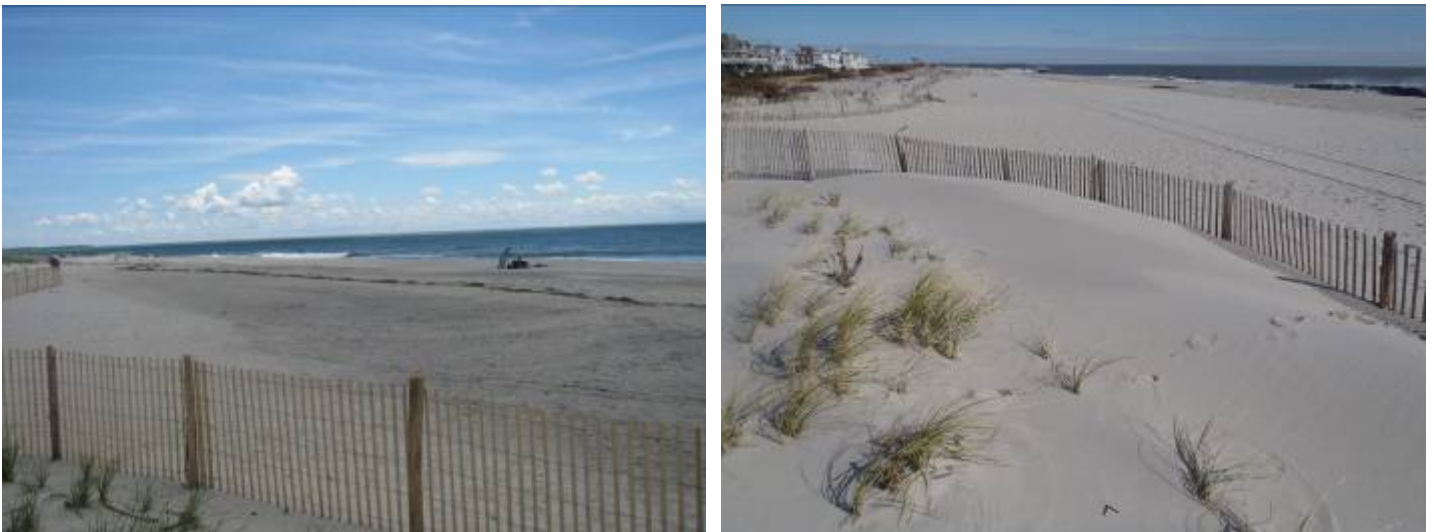
The left picture was taken in June 5, 2012 showing the beach toward the northeast. The post-storm shot on the right was taken November 9 th . The sand can be seen deposited around the fencing leaving only two rows of wire above the sand while in June there were 5 rows of wire showing. Here the beach was also widened toward the zero elevation position.
