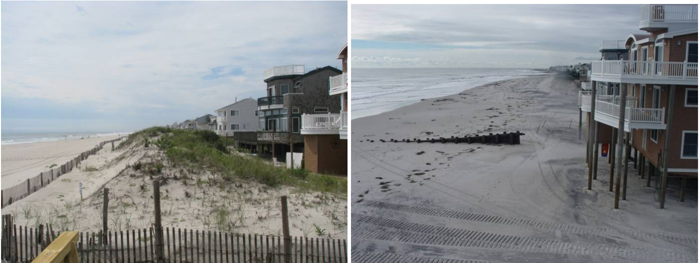
The photographs above were taken on September 6 th , 2012 (left) and November 1 st , 2012 (right). Both images show the view of Webster Avenue in Beach Haven (site 135) looking south. It is evident in the photographs that the existing dune was completely eroded away and overwash occurred, with waves pushing water and sand under the oceanfront homes and into the streets landward of them exposing the timber section of an old groin that was not exposed prior to the storm.
