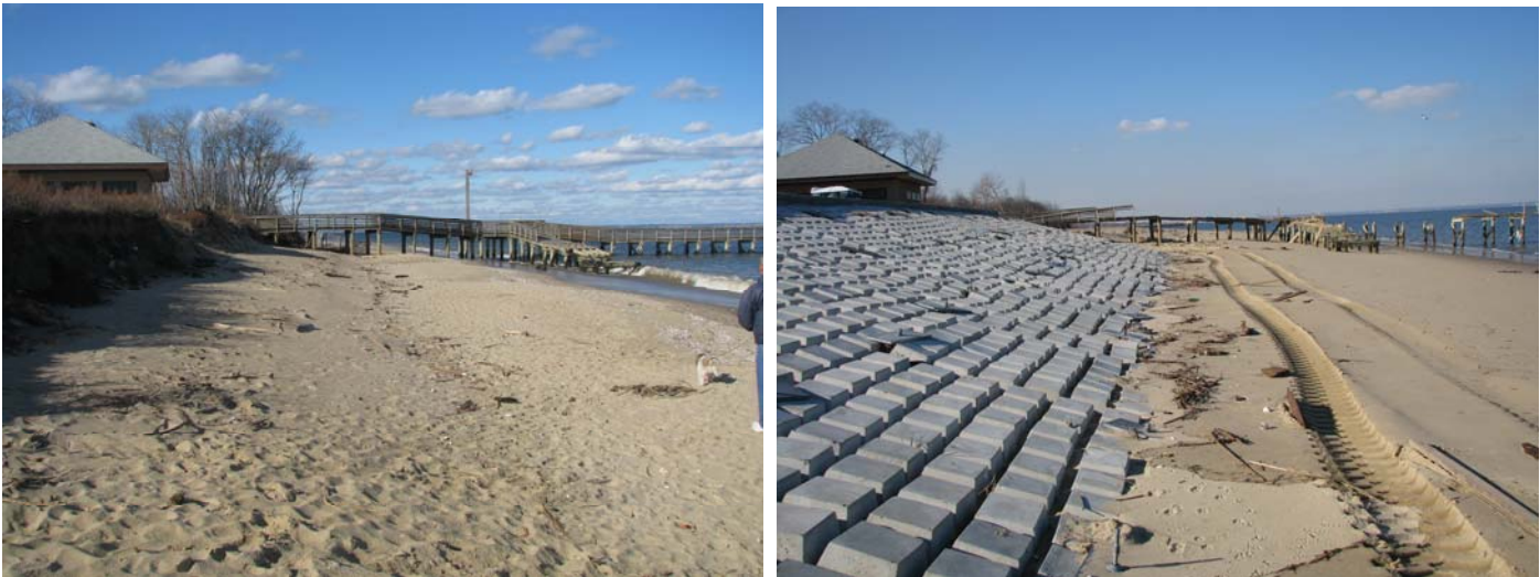
This site was damaged during H. Irene in 2011 which led to municipal efforts to harden the shoreline with an interlocking block revetment. The photograph on the left shows the shoreline on November 30, 2011. The photo on the right shows the revetment post Sandy (taken on December 13, 2012).
