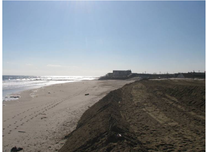
This site received sand during the Federal beach nourishment and maintenance projects (left photo taken May 30, 2012). This site was the most heavily damaged along the northern Monmouth County shoreline from Hurricane Sandy because there was a gap in the rock seawall and large grade-level pedestrian gaps in the small dunes (right photo taken).
