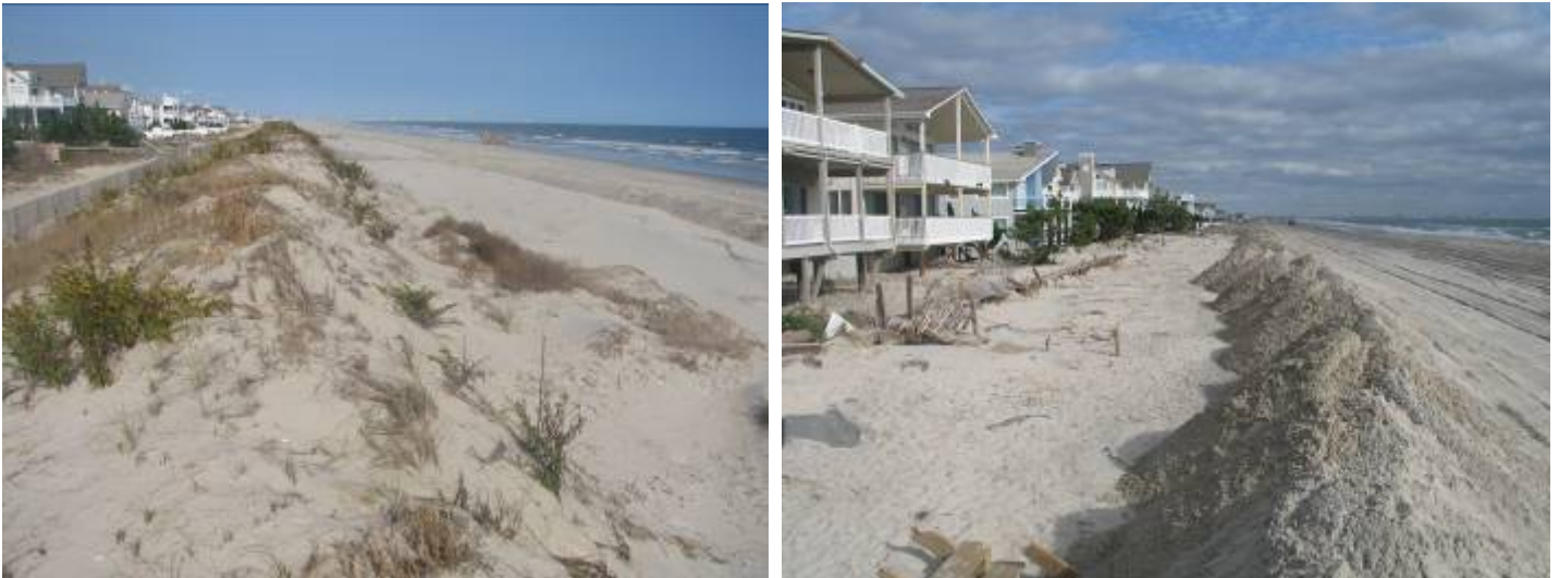
The left photograph was taken October 26, as Sandy was approaching NJ. Machines were deployed pushing up a ridge of sand seaward of the existing dunes at this site. Sandy overwhelmed the shore protection, jumped the old bulkhead and washed well inland producing damage and flooding. The right picture was taken November 6 th and shows recent bulldozing efforts to provide a small measure of protection for homes with nothing between them and the sea.
