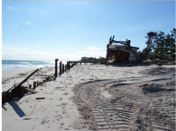
Pre-storm conditions of the modified dune are shown in the September 17, 2012 (left). This view shows the results of the restoration effort following Hurricane Irene (August 2011). The November 5, 2012 (right) was taken at the same location. This profile location is within 300 feet from the temporary breach that opened during Sandy. The home at 1117 Ocean Avenue was completely removed from its location and the residence in the photograph was also destroyed.
