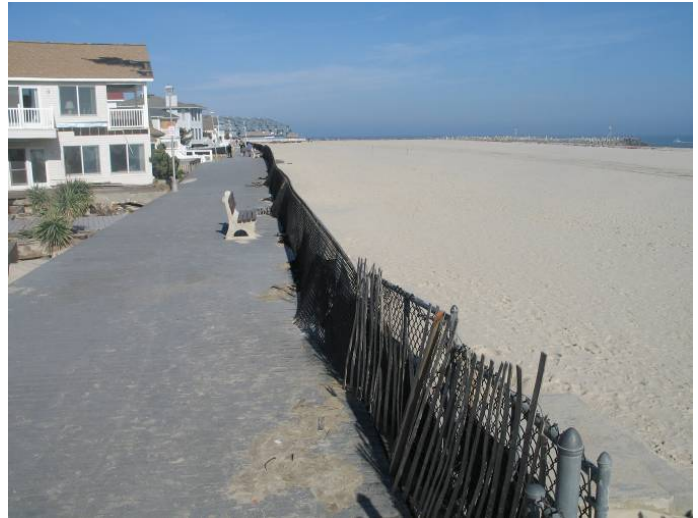
The photograph on the left was taken on September 21, 2012. The one on the right shows no noticeable change to the backbeach elevation following the storm (taken November 12, 2012). This urban beach did not have a dune system but was spared from more severe damages by the over 600-foot protective berm.
