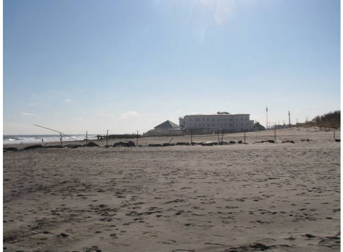
Low, wide dunes established naturally following the initial Federal beach nourishment project. Sand volumes have been relatively stable since that time (left photo taken March 22, 2012). Sandy’s storm surge and waves relocated sand from the dune and berm to both landward to the rocks and over the rocks, and to the nearshore (right photo November 21, 2012).
