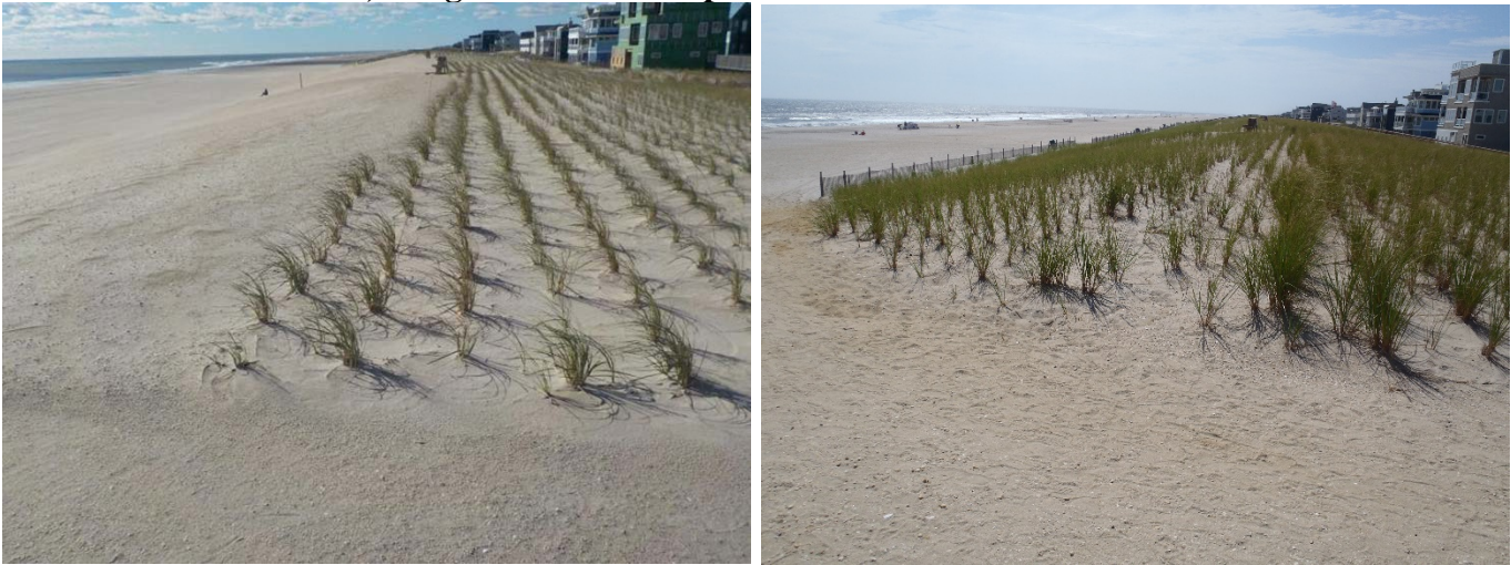
The 81 st Street profile in Long Beach Township received sand via federal beach fill in summer 2015 and planting of the dune vegetation was completed by fall 2017. The dune remained stable over the time period (left photo taken October 28, 2016 and right photo taken September 14, 2017, both views from the dune crest).
