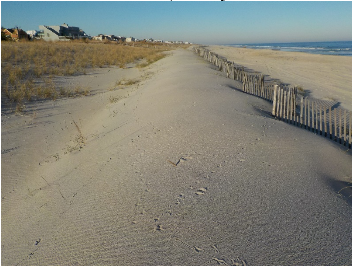
At the 73 rd Street profile, the engineered dune that was created in the 2009 federal beach fill remained in relatively the same position, though the seaward toe accumulated sand due to the presence of the sand fencing (left photo taken November 18, 2016 and right photo taken September 15, 2017).
