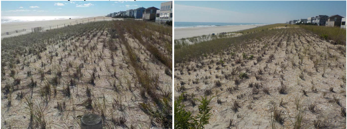
The photos from the dune crest at the Tranquility Drive location (left taken October 28, 2016 and right taken September 15, 2017) show no change in the engineered dune that was constructed in spring 2013.
