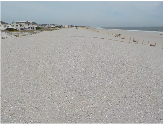
The Webster Avenue photos show the unvegetated and vegetated dune crest (left taken September 21, 2016 and right taken September 13, 2017). Some sand accumulated at the seaward base of the dune between fall 2016 and fall 2017 as a result of sand trapped by fencing.
