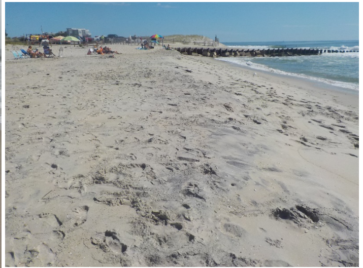
The photos above show the seaward portion of the berm immediately down-drift of the Holgate terminal groin (left photo taken September 21, 2016 and right photo taken September 13, 2017). The profile is located within the taper area of the federal beachfill.
