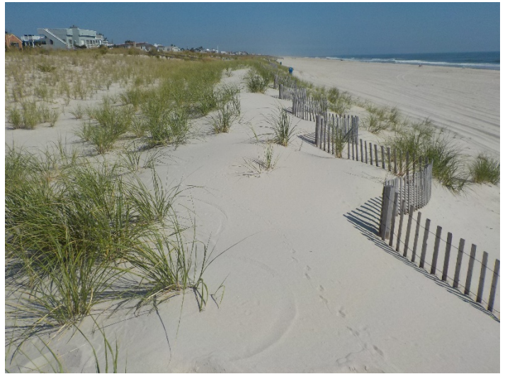
At the 73 rd Street profile, the engineered dune that was created in the 2009 federal beach fill remained in relatively the same position, though the seaward toe accumulated sand due to the presence of the sand fencing (left photo taken November 18, 2016 and right photo taken September 15, 2017).
