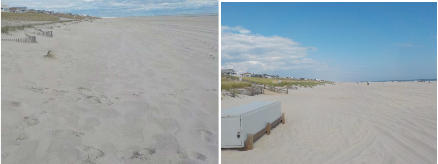
The Ship Bottom profile location has retained the dune position and a wide berm since the spring 2015 beach fill (left photo taken October 28, 2016 and right photo taken September 14, 2017).
