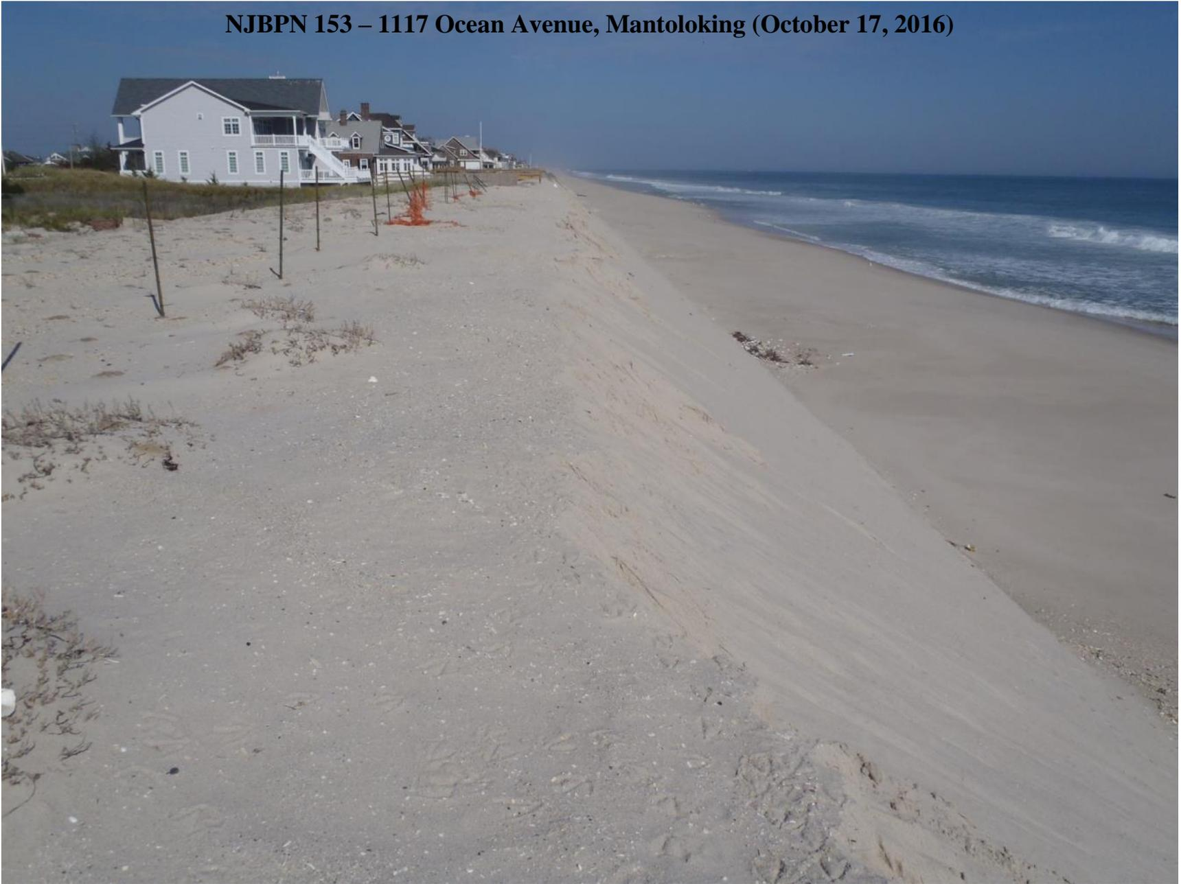
**Figure 238. View to the north from the top of the sheet-pile wall at 1117 Ocean Avenue in Mantoloking. The Borough conducted an extensive operation in bulldozing sand from the berm back to the steel wall following the northeast storm (Jonas) in late January 2016. This view shows the steep slope to the beach existing as of December 2016.**
