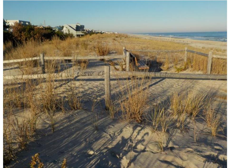
**Figure 323a & 323b. The photos show the condition of the vegetation on the engineered dune that was created in the 2009 federal shore protection project. Though scarped by Hurricane Sandy's waves, the dune (and wide beach) provided the necessary protection to landward properties during the storm. The 2013 emergency fill restored the dune and berm to the original design template. Left photo was taken September 15, 2015 and right photo taken November 18, 2016.**
