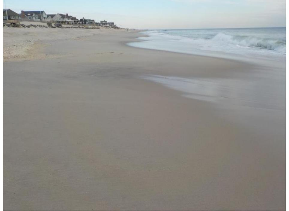
**Figure 233a & 233b. Both photos (left taken December 14, 2015 and right taken December 22, 2016) show the condition of the berm at the Bay Head location. The revetment rocks were covered just prior to Jonas on the left, but were exposed on the right 11 months later.**
