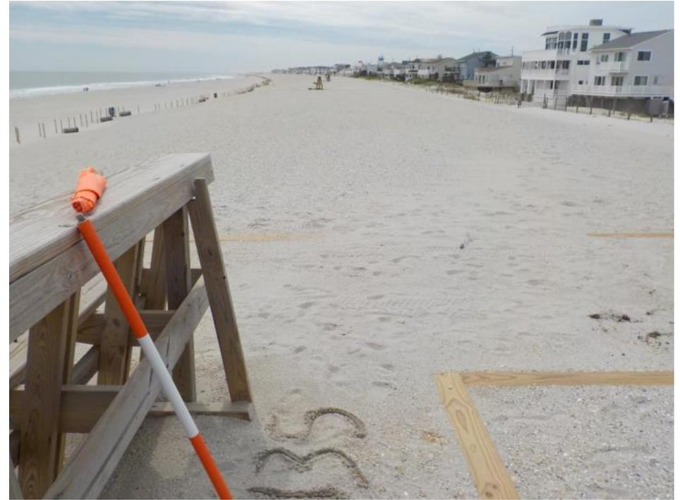
**Figure 377a & 377b. The photos show the view to the south from the dune crest at Webster Avenue. The left photo (taken December 15, 2015) shows the dune that was constructed in 2013 from sand that had been recovered following Hurricane Sandy. The right photo (taken September 21, 2016) shows the condition of the engineered dune prior to fencing and planting of vegetation. The engineered dune was constructed seaward of the 2013-2015 feature.**
