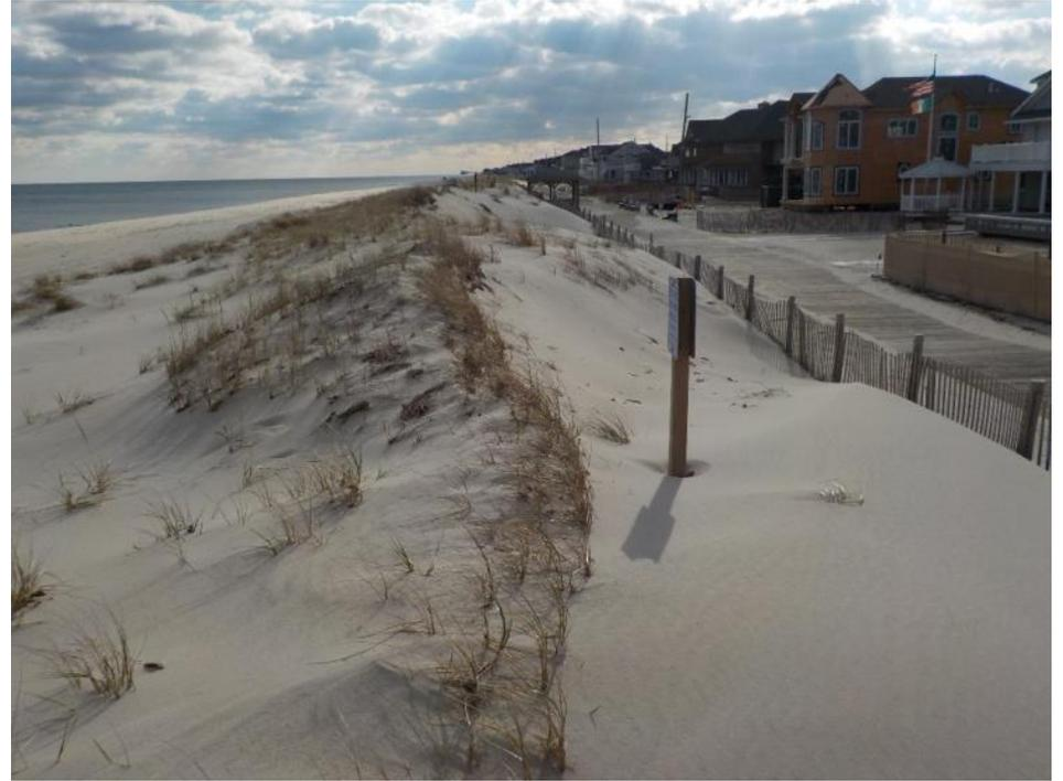
**Figure 257a & 257b.** The photos show the condition of the dunes at the Lavallette site (left photo taken December 11, 2015 and right photo taken December 9, 2016). Hurricane Sandy eroded the dunes at this site and these modest dunes were created from sand that was recovered after the storm. Some sand accumulated at the seaward base of the dune after the June 2015 survey.
