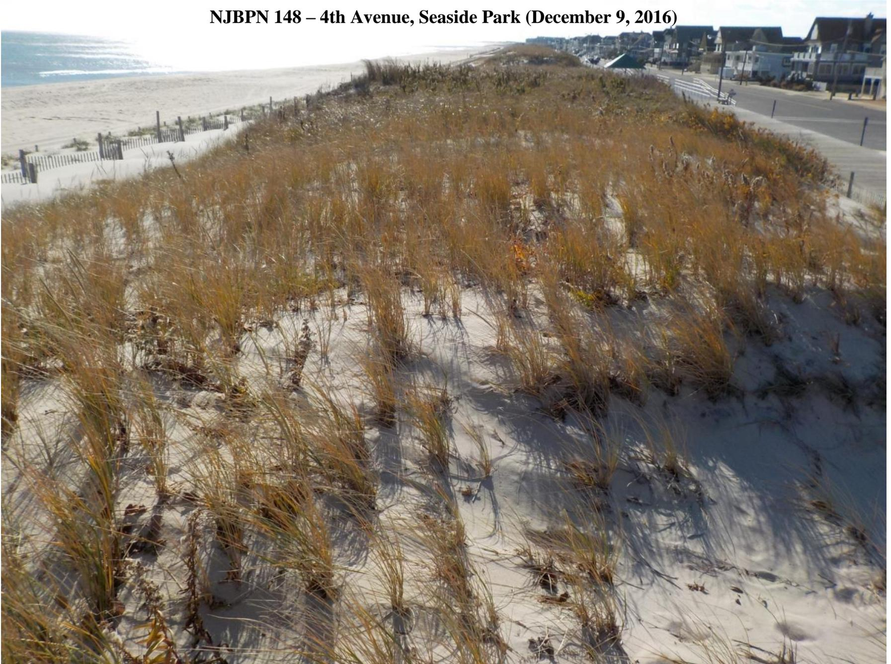
**Figure 274. View to the south from the dune crest at 4<sup>th</sup> Avenue in Seaside Park that show parking, dune condition, and new fencing partially buried by wind deposited sand.**
