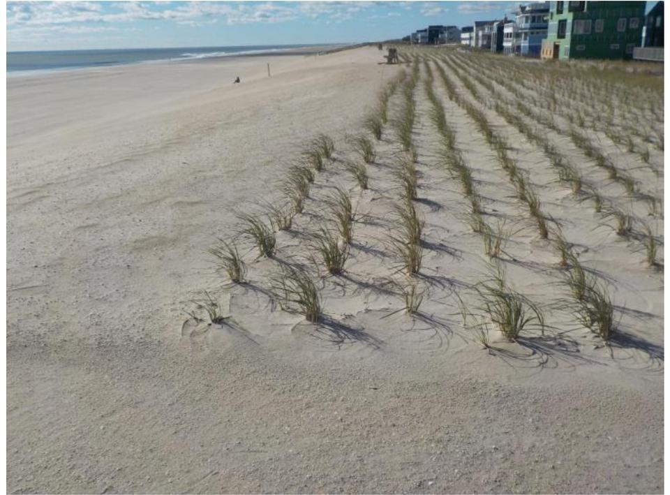
**Figure 353a & 353b. The view from the dune crest at the 81<sup>st</sup> Street location shows the newly constructed dune in 2015 (left photo taken December 15, 2015) and the dune with partially planted vegetation (right photo taken October 28, 2016). Sand fencing and more planting was set to be completed shortly after the picture was taken.**
