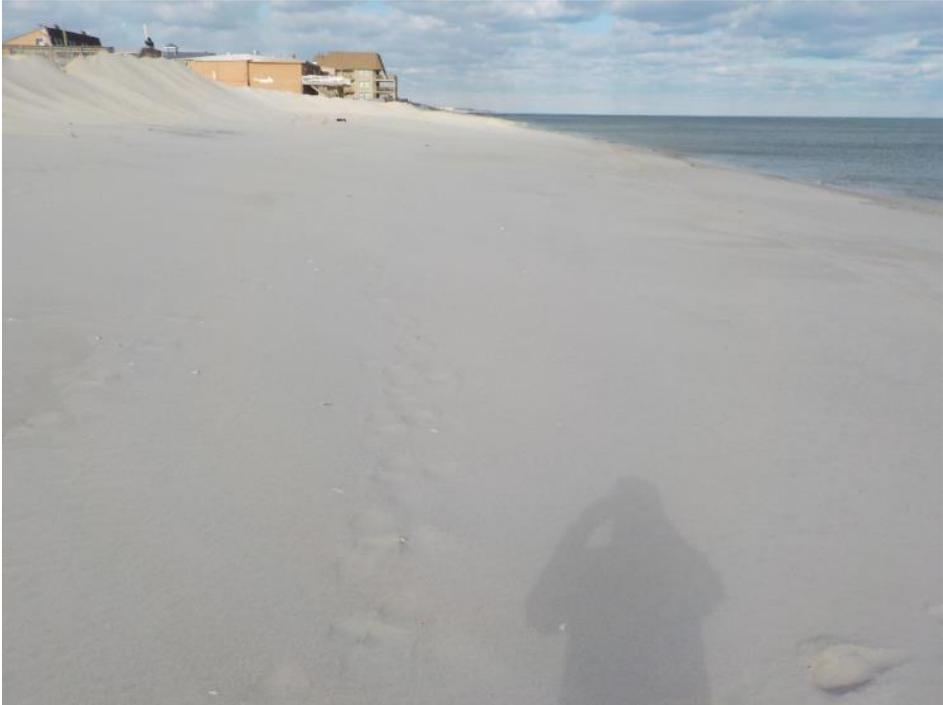
**Figure 263a & 263b. The photos show the condition and width of the berm at 8<sup>th</sup> Avenue in Ortley Beach (left photo taken December 11, 2015 and right photo taken December 9, 2016). Sand was added to reinforce the dune that was damaged during the January 2016 northeast storm.**
