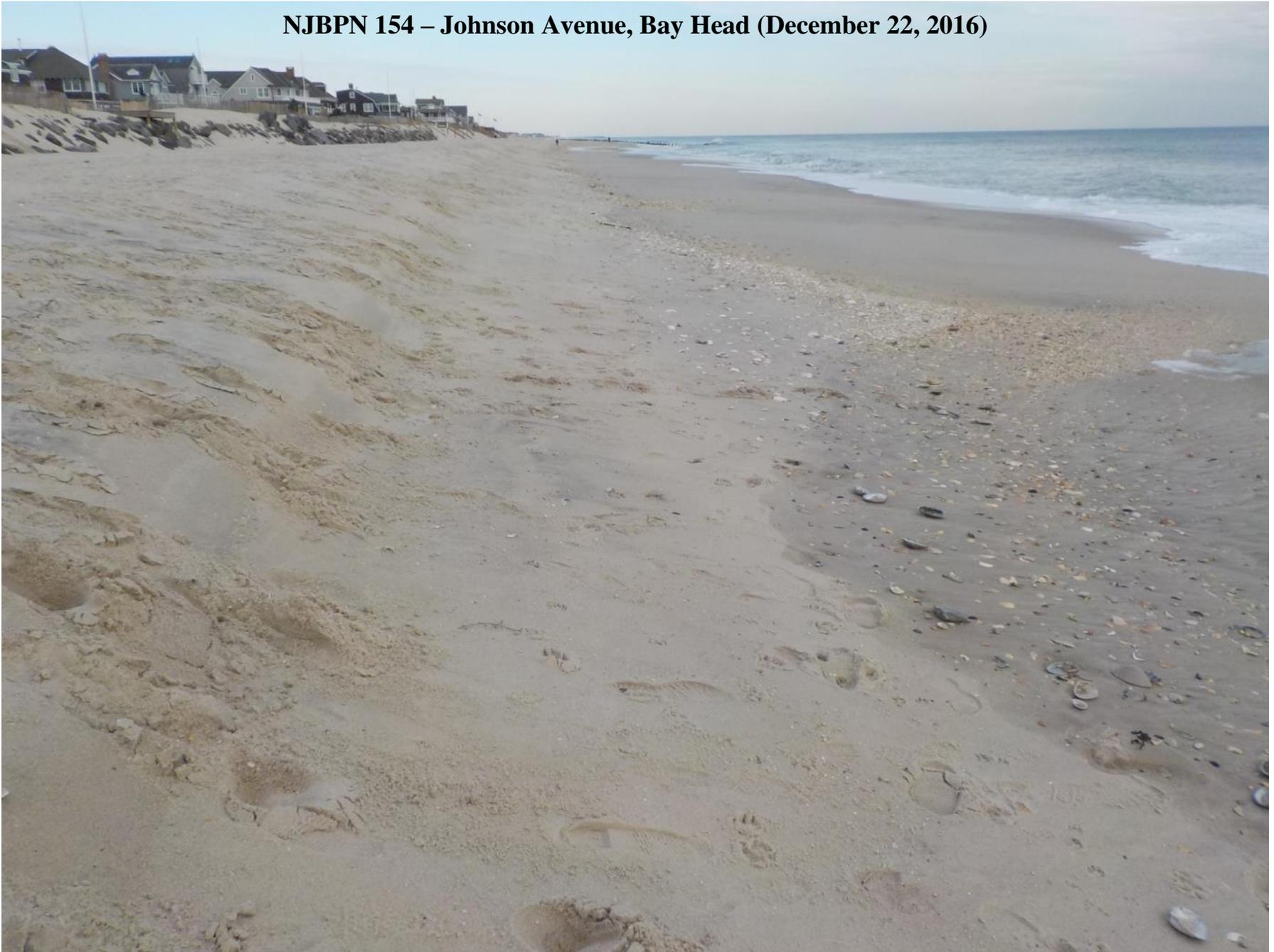
**Figure 232. View to the north from the berm break at Johnson Avenue in Bay Head. The rock revetment was exposed following the January 23, 2016 northeaster (Jonas). Here, the berm was eroded into a steep slope with waves reaching its base.**
