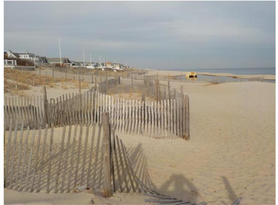
**Figure 227a & 227b. The Maryland Avenue profile is located over a mile south of Manasquan Inlet. The photos (left taken December 14, 2015 and right taken December 21, 2016) show a maintained beach. Installation of sand fencing seaward of existing fence is a local effort to capture wind-blown sand. The stormwater discharge station from Sea Avenue is evident on the right photograph, but not so visible on the left.**
