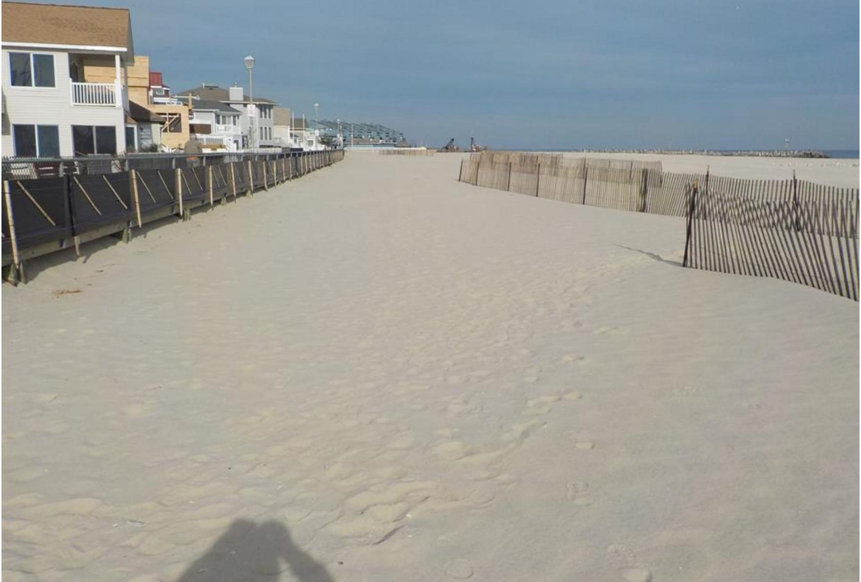
**Figure 219. View to the north from the backshore at Water Street in Point Pleasant Beach. The en eschelon rows of sand fence could be the locus of a dune along this section of beach. Any dune over 4 ft high would have prevented the overwash that was experienced during Hurricane Sandy.**
