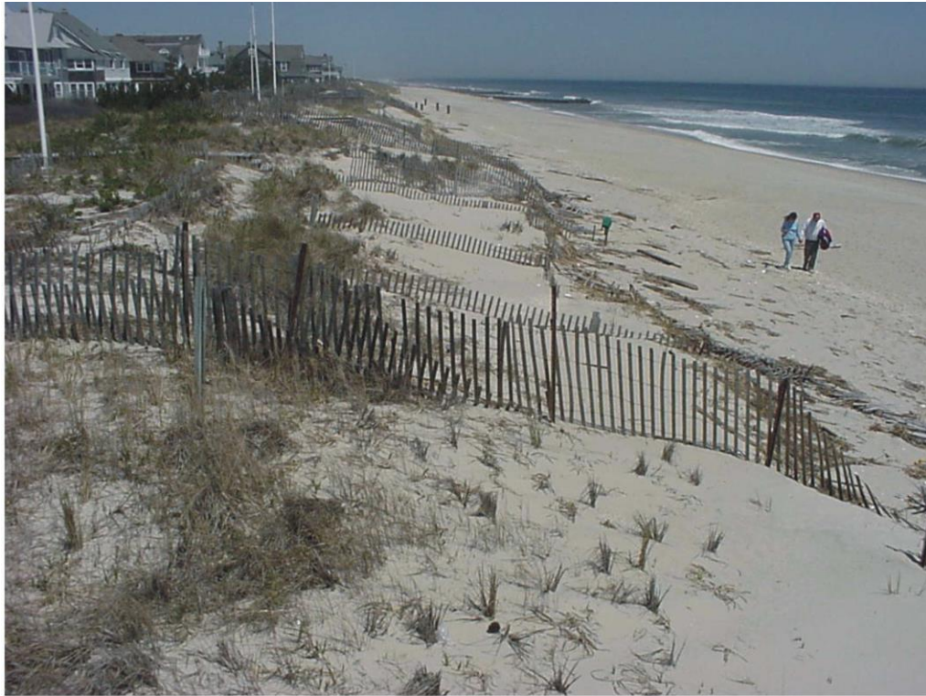
Photoplate 3a. Photo taken April 28, 2003 looking north from Johnson Street in Bay Head. Dune grass plugs show in the foreground prior to growth in the spring. Winter storm damage shows in broken dune toe fencing placed low on the slope where wave action easily reached the fragile fence.
