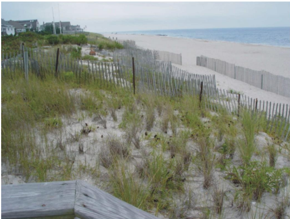
Photoplate 3b. In this photo taken August 30, 2004, a year and a half later. The dune grass plugs survived, but did not flourish. The vegetation across the dune did increase in quality however. The fence at the dune toe is again placed where it will be easily destroyed by any type of storm. Placement a third of the distance up the seaward slope is recommended.
