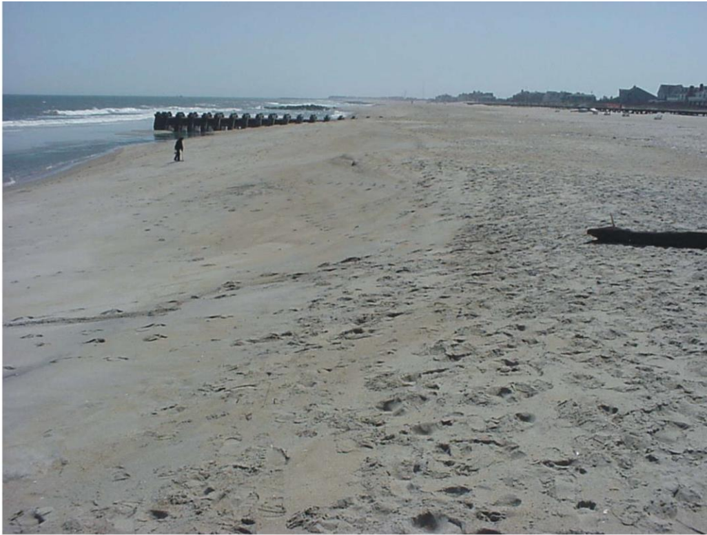
Photoplate 2a. Looking south from New York Ave. in Sea Girt, NJ with a stormwater outfall pipe emerging from the berm onto the low tide beach. The beach between the berm crest and the boardwalk is the result of the ACOE fill project along this shoreline. The picture was taken April 15, 2003
