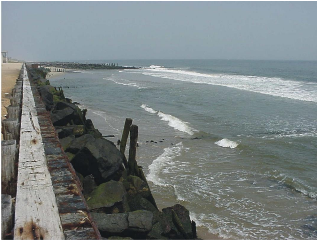
Photoplate 1a. This photo was taken on May 31, 2000 at NJBPN 171 (Pullman Avenue, Elberon). Although following the ACOE fill project by several years, the sand quantity present here remained insufficient to produce even a low-tide sand beach.
