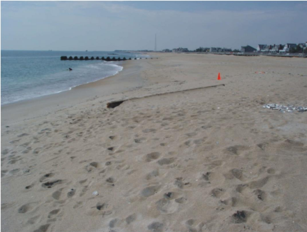
Photoplate 2b. By April 8, 2004 minor berm retreat has exposed only one more piling support section on the outfall pipeline. The shoreline retreated 1.2 feet during the time interval, as measured at the profile line (#159), with a sand volume gain of 14.6 cubic yards.
