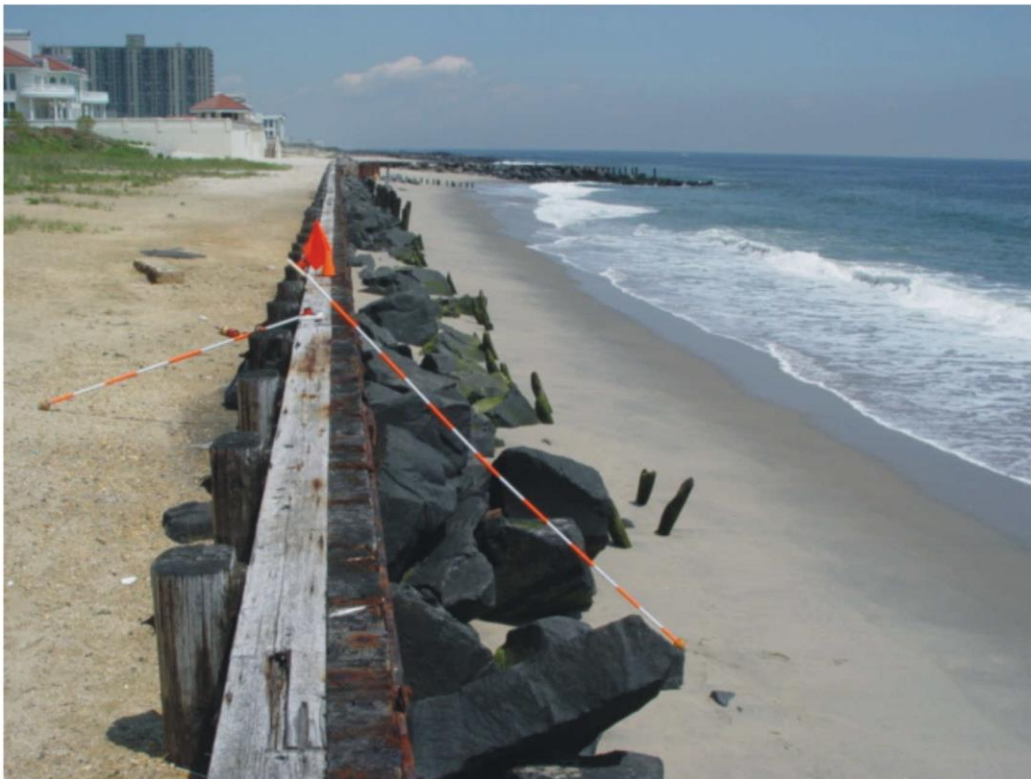
Photoplate 1b. By June 3, 2004 the site showed a substantial sediment accumulation allowing a beach at the rocks almost above the level of most high tides. This process has not been continuous with growth seen every six months between surveys, but the conclusion is that this material comes from Long Branch.
