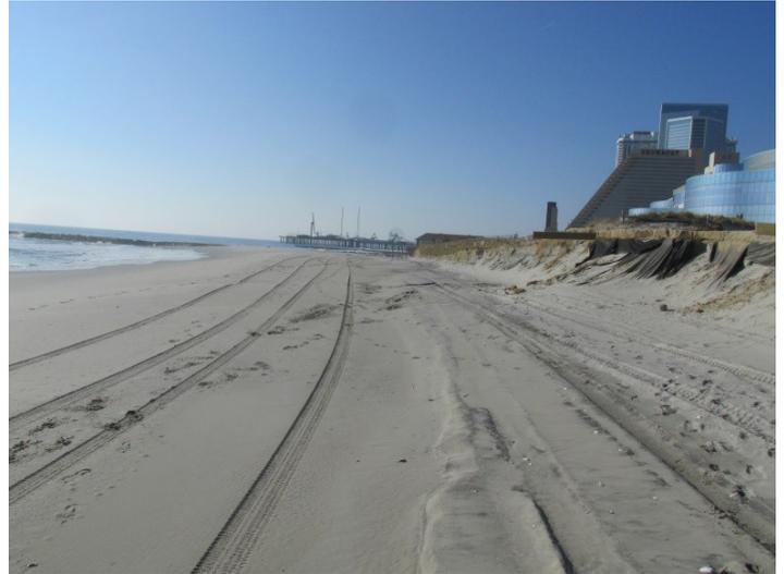
This profile site is located near the Absecon Inlet south jetty. The December 4, 2014 (left, view to the south) shows a scarp cut into the back beach just short of the dune fencing. The right photo (taken December 10, 2015) shows that the fencing is gone and the dune itself has been compromised somewhat by shoreline retreat.
