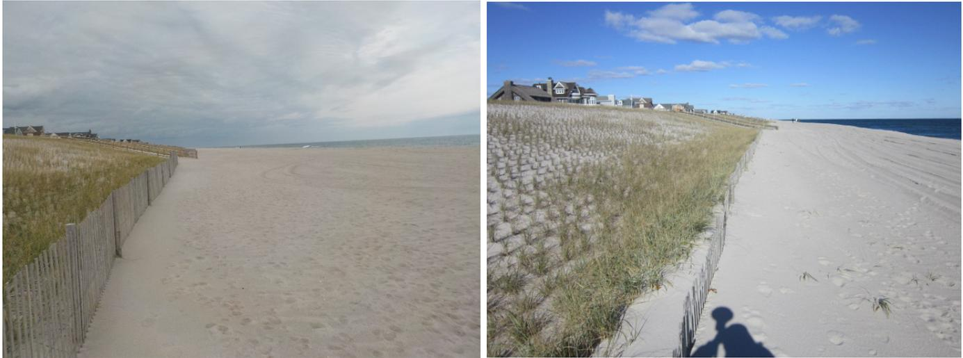
The photos of the Normandy Beach profile show the conditions of the seaward dune toe of the engineered dune that was completed in December 2018 (left photo taken November 5, 2019 and right photo taken November 18, 2020). The fall 2020 photo and profile show sand accumulated at the fence.
