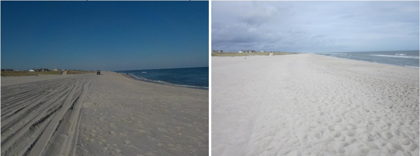
The photos of the 6<sup>th</sup> Lane location (left November 5, 2019 and right taken November 11, 2020) show the conditions of the berm since completion of the beachfill that occurred in February 2019. The seaward portion of the berm gained in elevation between spring 2019 and fall 2020.
