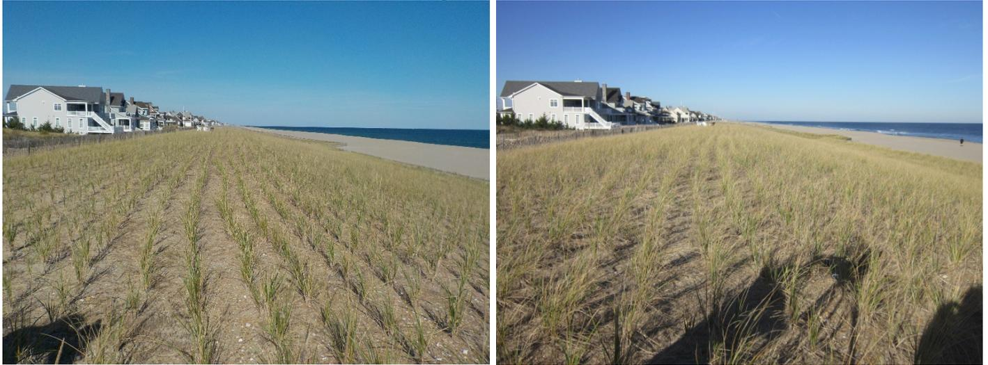
The photos of the 1117 Ocean Avenue profile show the condition of the engineered dune that covers a steel bulkhead that was constructed in 2015 (left photo taken November 4, 2019 and right photo taken November 20, 2020). The dune remained stable over the 2019-2020 time period, but berm width decreased. The 0.0 ft NAVD shoreline moved landward (-46.25 ft) from its fall 2019 position.
