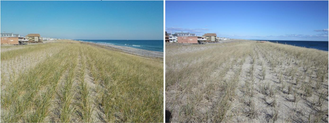
The Ortley Beach photos show conditions on the engineered dune that was completed in November 2018 (left photo taken November 6, 2019 and right photo taken November 18, 2020). Over 2019-2020, the 22 ft high dune remained in position and elevation.
