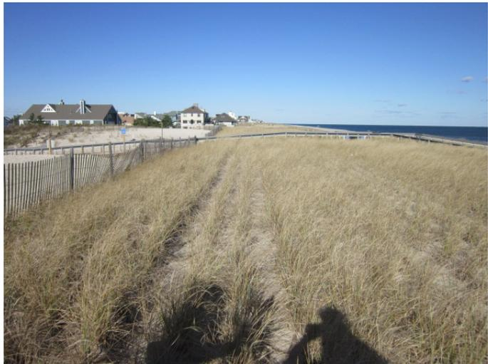
The beachfill was completed at the Brick Township Public Beach #3 profile site in summer 2018 with the engineered dune covering the steel bulkhead. The photos show the condition of the dune (left taken November 5, 2019 and right taken November 18, 2020). The dune remained in position and elevation throughout 2020.
