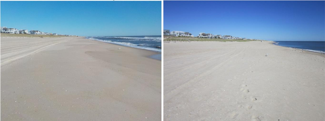
A supplemental beachfill was completed at the 20<sup>th</sup> Street profile in July 2018. By fall 2019 (left photo taken November 1, 2019) berm width was within 25 feet from the fall 2018 position. In fall 2020, berm width was similar to fall 2019 (right photo taken October 8, 2020).
