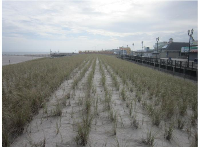
At the Franklin Avenue profile, an engineered dune was constructed within the federal beachfill in January 2019. No dune existed prior to the beachfill. The dune remained stable through 2020 (left photo taken November 6, 2019 and right photo taken November 11, 2020).
