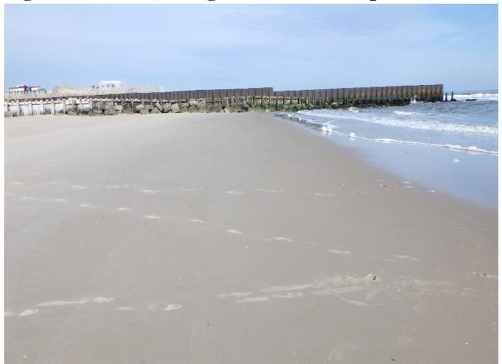
The Holgate profile lies 200 feet downdrift of the Holgate terminal groin and the photos show the changes near the swash zone (left photo taken September 9, 2019 and right taken September 25, 2020). Berm widths and sand accumulations have been highly variable through the 26 years of profile monitoring largely due to large differences in sediment supplies passing the terminal groin onto this beach.
