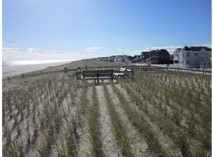
The left photo (taken November 5, 2019) shows the engineered dune which was created from the integration of sand recovered from Hurricane Sandy and the beachfill that was completed at this location in April 2019. The right photo (taken November 18, 2020) shows planted vegetation on the engineered dune.
