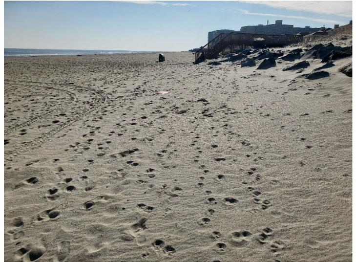
This site was the southern location within Phase I of the federal project. On the left, the rock wall was partially buried in wind-transported sand (Jan 16, 2020). The right-hand view on Jan. 12, 2021 shows the rock toe of the revetment further buried in wind-deposited sand.
