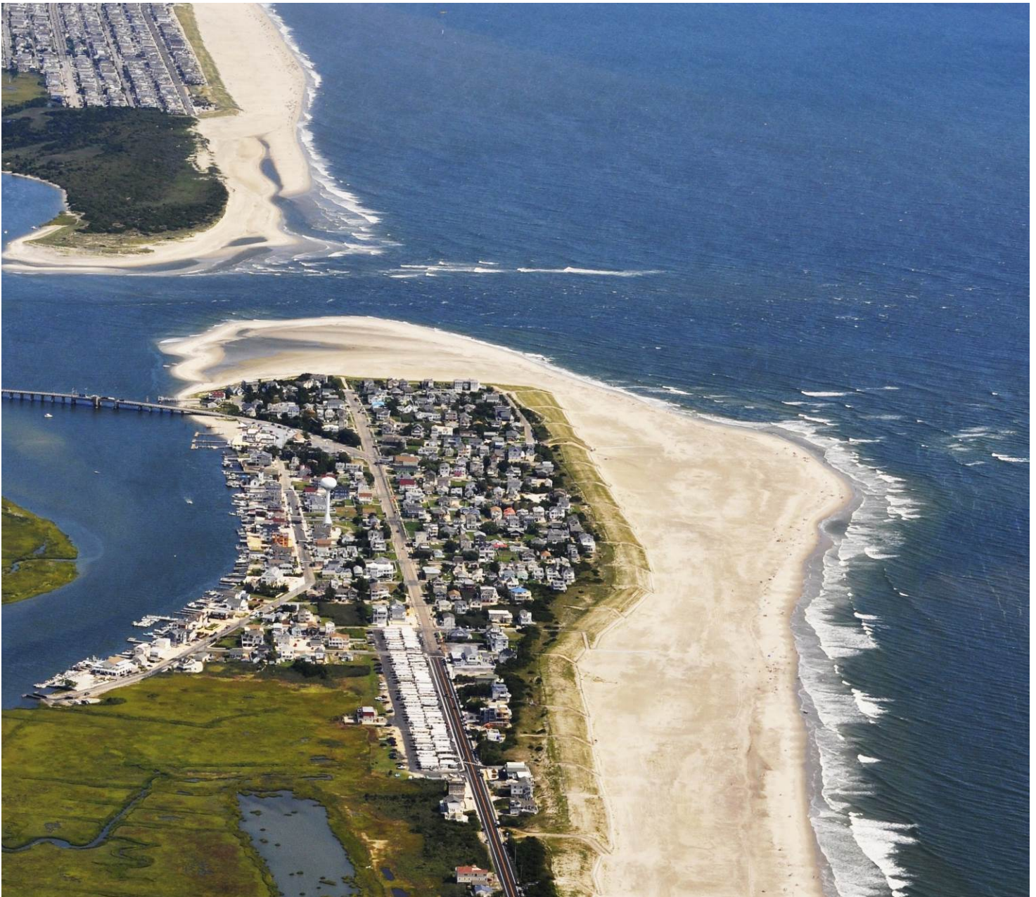
Figure 15. Aerial photograph taken September 2, 2016 by Ted Kingston looking north, northeast across the wide central beaches of Strathmere showing where sand is accumulating in the zone between Williams and Tecumseh Avenues as a pronounced lobe extending several hundred feet seaward of the average shoreline trend. The sand coming south from Ocean City is clearly present as the long spit reaching the inlet as a barely submerged shoal. The northeast Strathmere shoreline has assumed a northeast perpendicular straight line shape signifying both wave and tidal current effects. Flood tidal currents do bring sand along this straight segment so long as the lobe remains in place with shoals to the seaward of it. The tidal currents in the inlet also show clearly as a straight-out exit for the moment.
