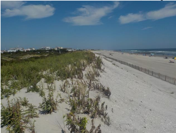
Photoplate 8a - Photo taken September 14, 2016 showing sand fence at the seaward dune toe. The profile shows a summer accumulation of sand on the berm.
