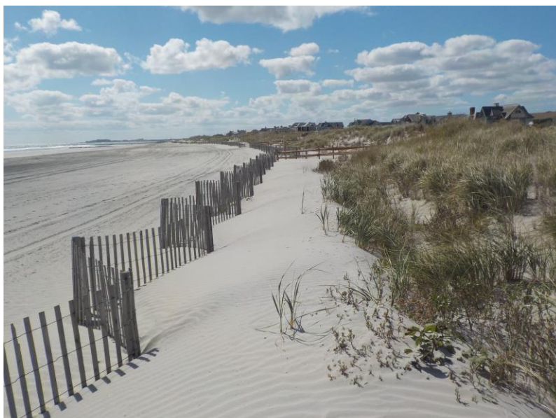
Photoplate 7c – Photo taken October 3, 2017 shows sand trapped by the sand fencing. This management practice allows the dunes to progress seaward.
