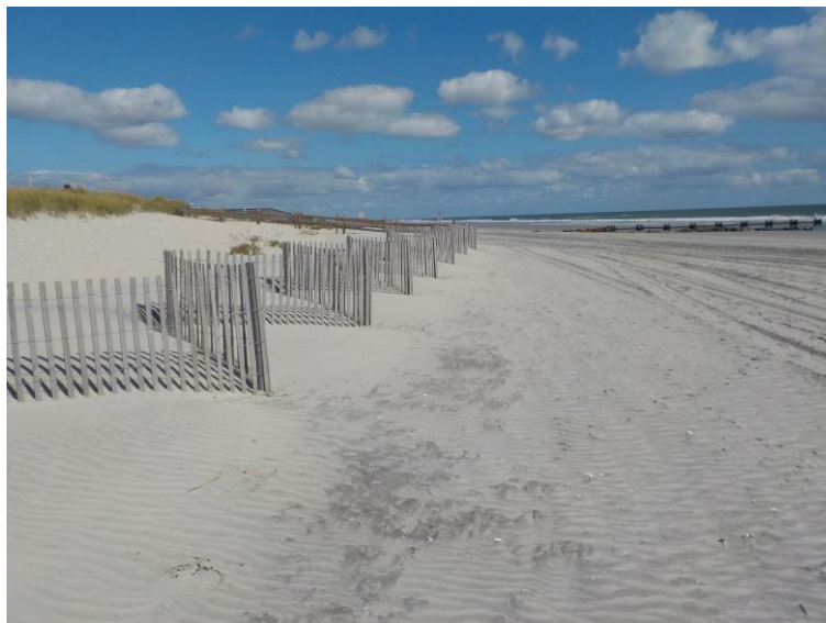
Photoplate 6c – Photo taken October 3, 2017 shows sand fencing at the seaward dune toe. The shoreline moved 29 ft. seaward from its March position.
