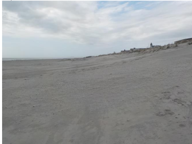
Photoplate 5b – The photo taken March 27, 2017 shows the wide berm from sand placed in the February-March beach fill.
