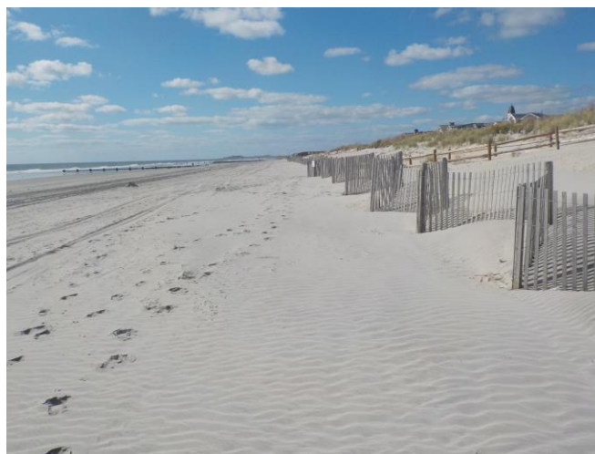
Photoplate 5c – Photo taken October 3, 2017 shows sand fencing to protect the seaward dune toe. The wide berm had reduced in size and elevation from its March position.
