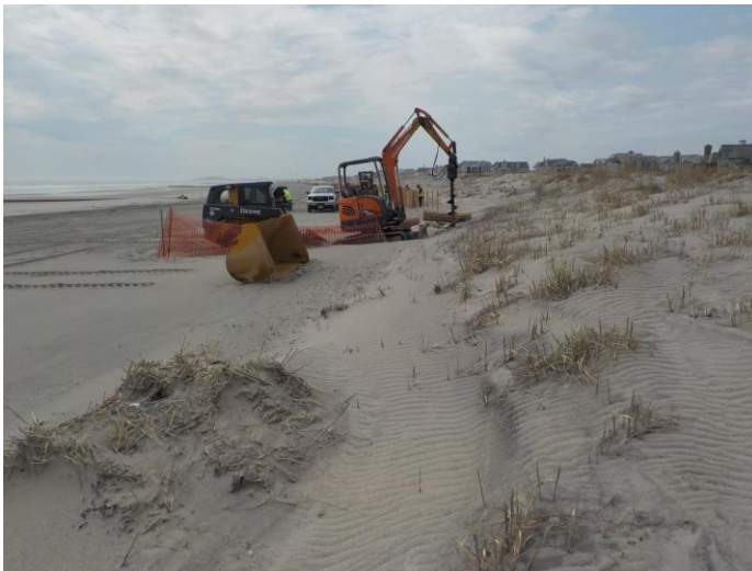
Photoplate 7b – Photo taken March 27, 2017 showing the installation of fencing at the toe of the dune.
