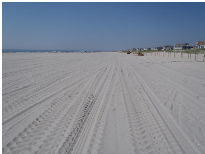
Photoplate 4b - Photo taken June 12, 2017 shows the southern limits of the north end beach fill. The beach width gained 200 ft. from its October 2016 position.
