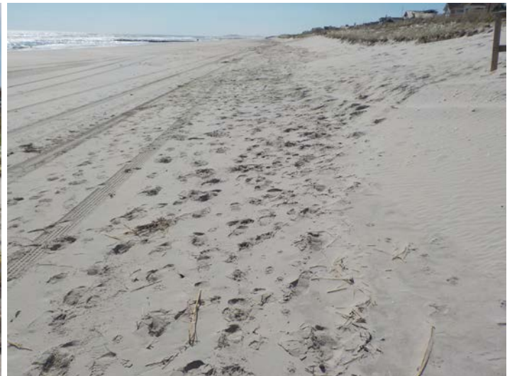
Photoplate 4b - Photo taken October 13, 2016 looking along the seaward dune toe location. The berm regrew and some sand was added to the dune toe making up for Jonas's erosion.
