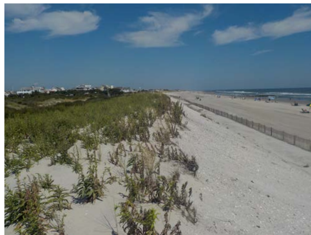
Photoplate 8b – Photo taken September 14, 2016 a few days after Hurricane Hermine passed the coast. The scarp has muted due to sand sloughing off the crest and wind deposition at the toe. A new sand fence was added and has started sand capture. There is a bar on the beach as a result of summer accumulation of sand.
