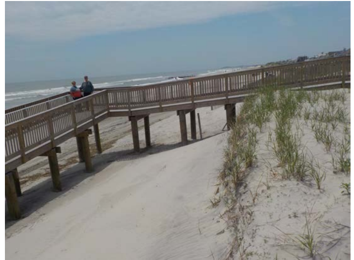
Photoplate 3b – By May 24, 2016 the dune scarp had blended into the seaward slope again, but the loss under the access ramp is still clear from the edge of the grass outward.
