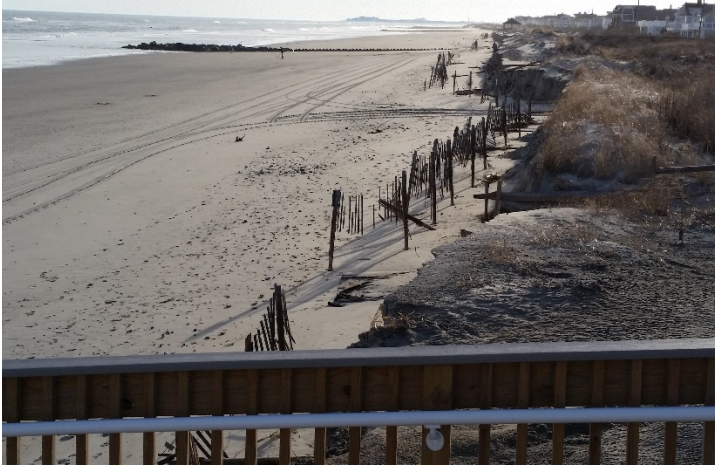
Photoplate 3a - Photo taken January 25, 2016 following Jonas. The access ramp was undercut and exposed. The last segment of the railing was gone, otherwise the structure was fine. The dune fencing was destroyed in both directions with 25 feet of seaward slope erosion beyond the fencing position.
