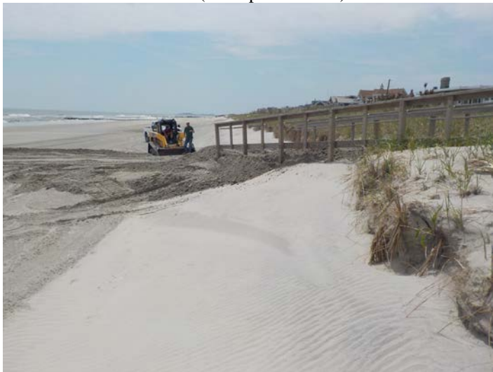
Photoplate 4a - Photo taken May 24, 2016 showing grading work taking place around the access pathway. There was erosion at the dune toe during Jonas that slowly recovered as sand was blown toward the dune from the beach.
