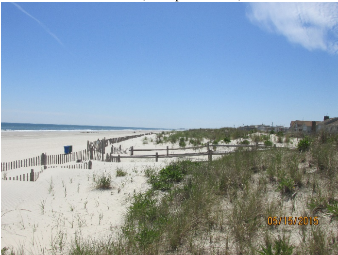
Photoplate 2a - Photo taken May 15, 2015. View to south along the row of dune fence from 90 th Street. Aeolian sand had begun to accumulate around the base of the fence, filling in to expand the seaward dune slope.
