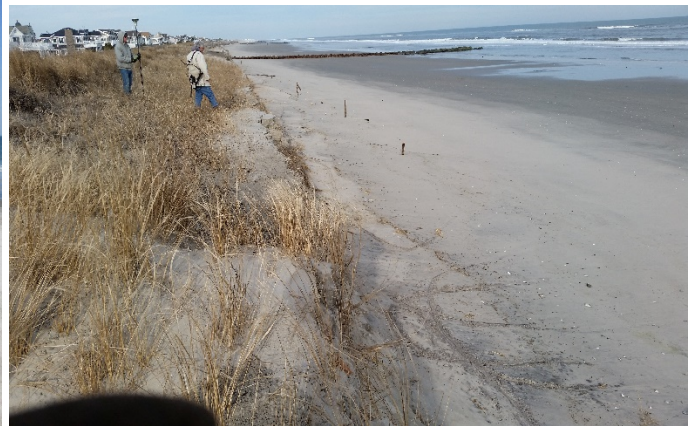
Photoplate 8b – Photo taken January 25, 2016 following Jonas. The scarp was 8 to 10 feet high and the seaward dune toe was cut back to within 20 feet of the bench up to the crest. The beach was flat and wet to the toe on the last high tide.
