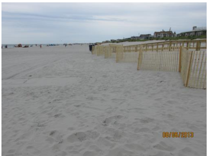
Photoplate 4b - Photo taken August 6, 2013 (spring 2013 survey [40]). View to the south along the dune toe from 103 rd Street. The 2013 USACE beach maintenance project restored the beach width and elevation to the original design template. Sand was placed on the seaward dune slope and a row of dune fence was installed to trap windblown sand.
