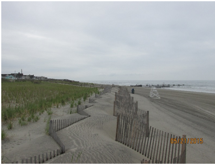
Photoplate 6a - Photo taken May 21, 2015. View to north along the dune toe from 112 th Street. The beach was narrow but wind-blown sand accumulated on the seaward dune slope.
