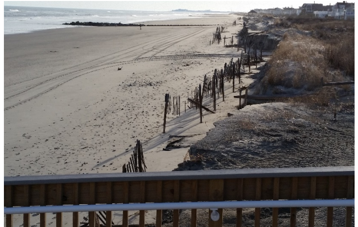
Photoplate 3b - Photo taken January 25, 2016 following Jonas. The access ramp was undercut and exposed. The last segment of the railing was gone, otherwise the structure was fine. The dune fencing was destroyed in both directions with 25 feet of seaward slope erosion beyond the fencing position.
