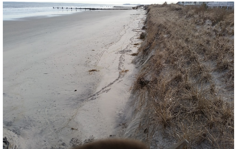
Photoplate 5b - Photo taken January 25, 2016 showing the dune scarp at 108 th Street looking south along the cut. The beach was wet to the toe of the scarp from the last high tide. Two weeks later additional erosion took place. All the dune fencing was destroyed with the storm taking all the recent deposition as well.
