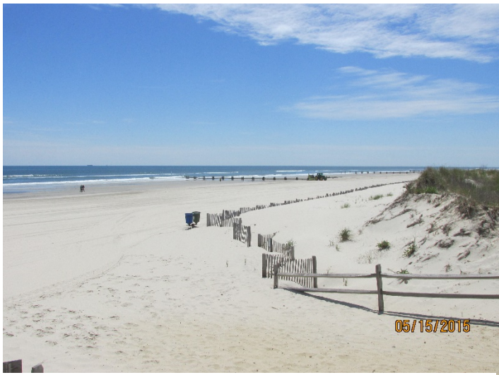
Photoplate 1a - Photo taken May 15, 2015. View to south along the dune toe from 82 nd Street. The dune fence installed after the ACOE project to capture aeolian sand had almost filled, but the beach remained relatively narrow.
