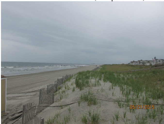
Photoplate 5a - Photo taken May 21, 2015. View to south along the dune toe from 108 th Street. Wind-blown sand accumulated on the seaward dune slope.
