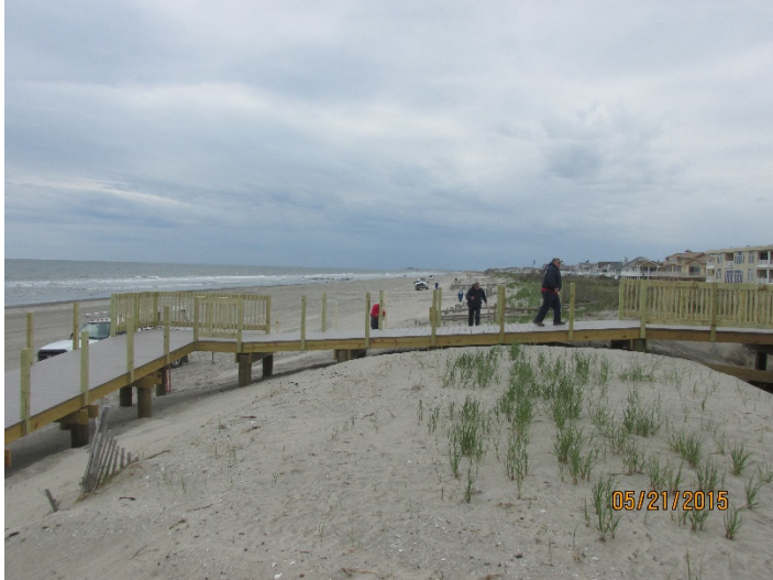
Photoplate 3a - Photo taken May 15, 2015. View to south along the dune toe from 95 th Street. A new access ramp featuring ADA access was built and withstood the Jonas storm. The erosion into the dune approximates where the individual standing at the edge of the grass is positioned in the photograph.
