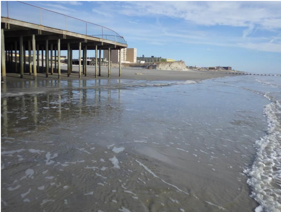
Figure 20. A view of the dune looking to the north from the shoreline located near 23 rd Avenue on November 3, 2016. The low lying recreational beach and absence of a protective berm has rendered the dune vulnerable to wave approach. Notice the large scarp in the dune located to the north of the pier. This dune was initially designed to extend to points seaward of the timber pier and extend south past all the pier structures. This design was mandated by the Land Use Regulatory agency of the NJDEP. It failed to survive storm events and was re-positioned at a point parallel with the shoreline at the existing scarp.
