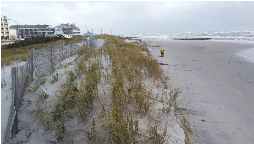
Figure 5. View from 5 th Avenue looking north taken on October 3, 2015 following the northeast storm events and Hurricane Joaquin. A significant scarp in the seaward dune face is shown along with recreational beach elevation and shoreline losses observed.
