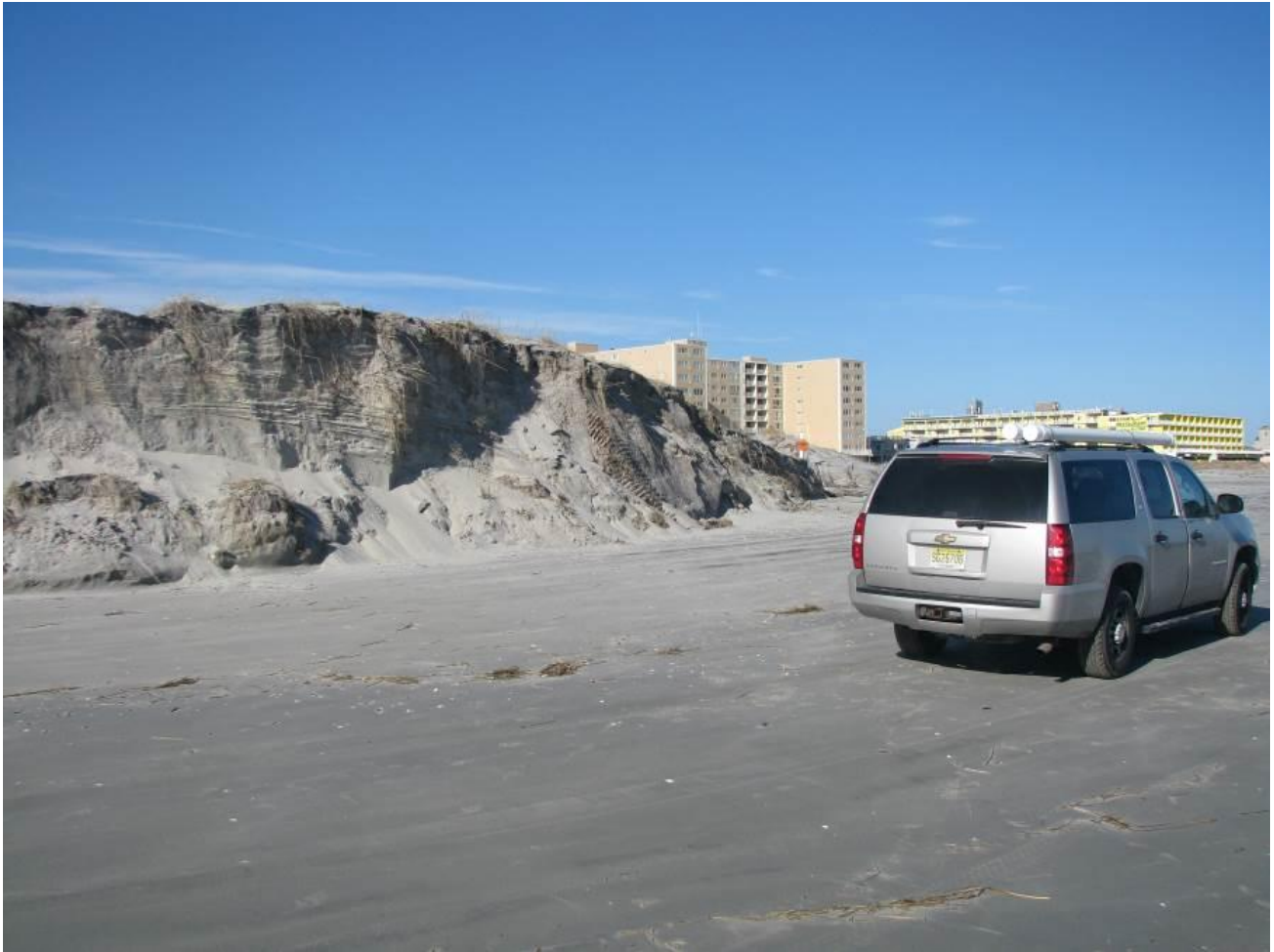
Figure 27. A close up view of the dune looking to the north from the beach located near 22 nd Avenue on January 27, 2016. Jonas caused severe erosion to the dune where a large scarp can be seen.
