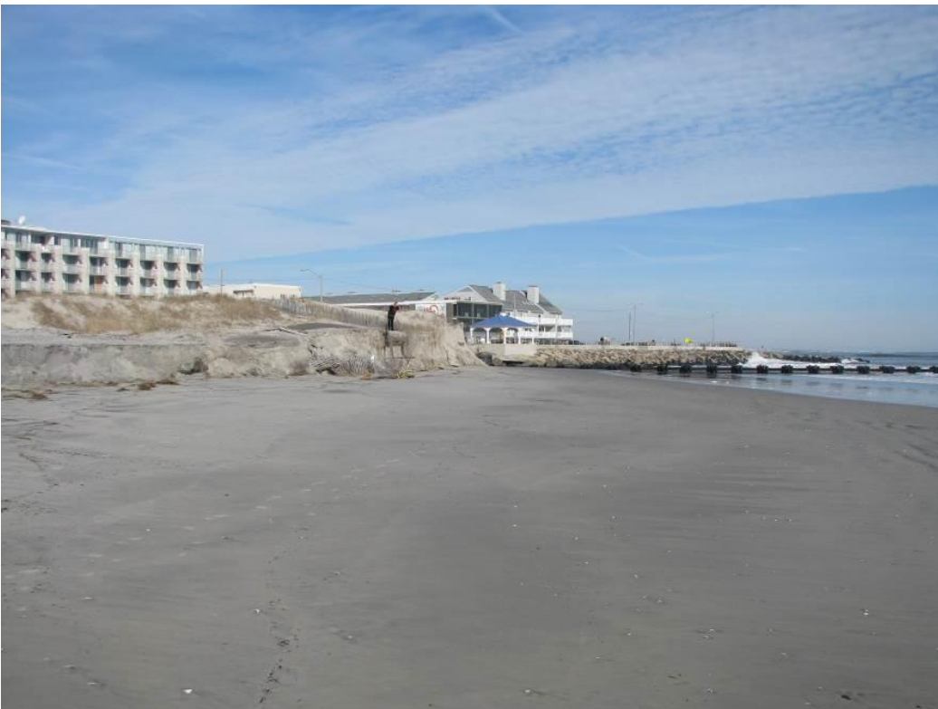
Figure 26. View to the north following Jonas taken at 5 th Avenue on January 25, 2016. The storm caused severe erosion to the beach and dune system creating the large scarp seen in the dune and the remainder of the sand from the Beach Creek dredge material pile.
