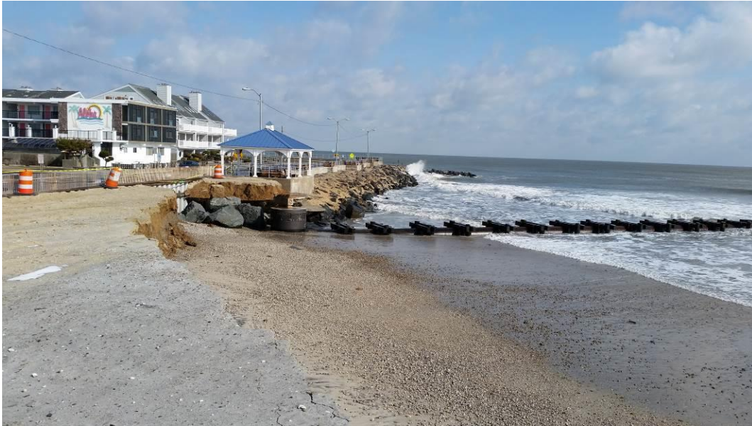
Figure 6. View from 4 th Avenue looking north taken on February 10, 2016. The primary dune and beachface has suffered severe erosion in the form of a large scarp. The gazebo and manhole access cover to the storm outflow pipe is completely exposed and extremely vulnerable to wave approach.
