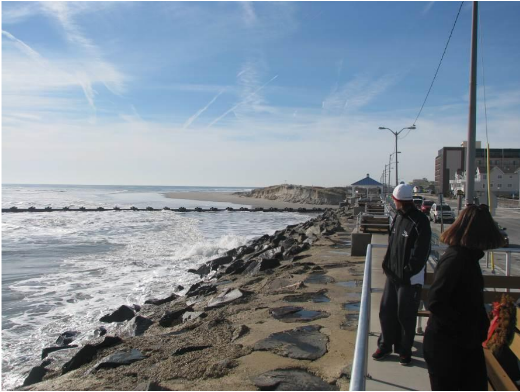
Figure 25. A close up view of the exposed seawall looking to the south at 2 nd Avenue on January 25, 2016. Winter Storm Jonas eroded sand in this area completely exposing the wall at virtually all stages of the tide cycle.
