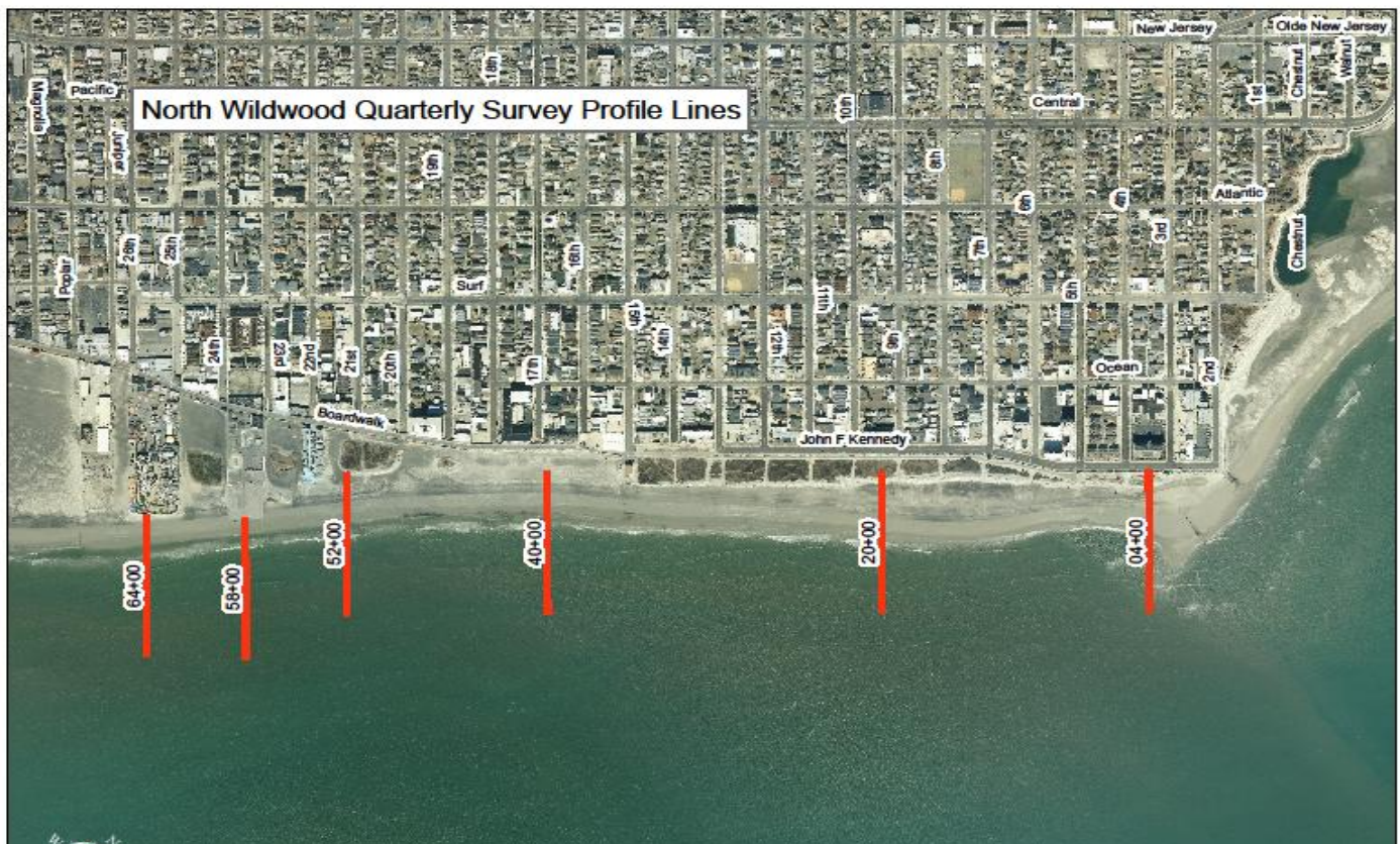
Figure 1. Shown above are locations of six representative profile sites of the 54 profile stations where shoreline changes were measured on the City’s oceanfront from October 2015 to November 2016. For each of the six profile stations descriptions and cross sections are provided to show typical changes over the year.
