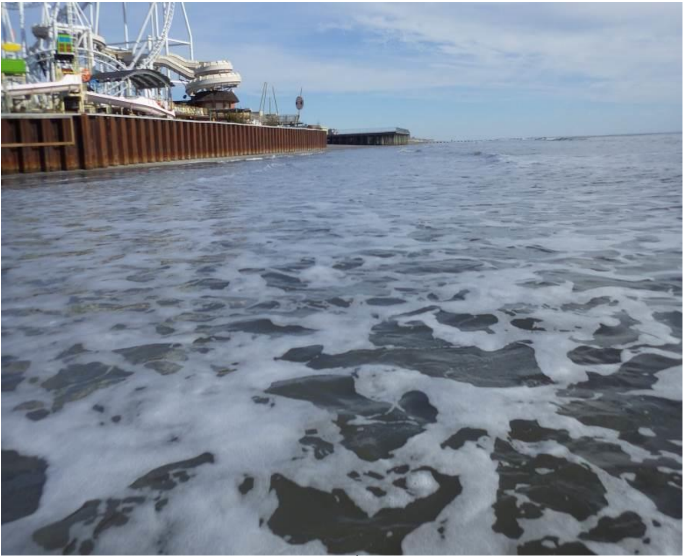
Figure 23. View to the north taken on February 12, 2016 near 26 th Avenue following winter storms Jonas and Nacio. The dry beach that was present less than two years ago has been eroded, leaving the ocean waves lapping at the base of the pier's steel bulkhead walls.
