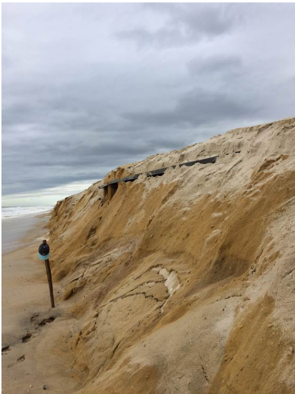
Site #6 located at Herbert Street shows the impacts of Hurricane Hermine to the left and the results on Nov 30, 2016 following a 3-day duration storm in late September.
