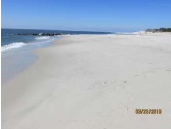
The 2015 photo taken on March 23 shows the offset in beach width and berm elevation between Coral and Lake Avenue beaches along the Coral Avenue rock groin.
