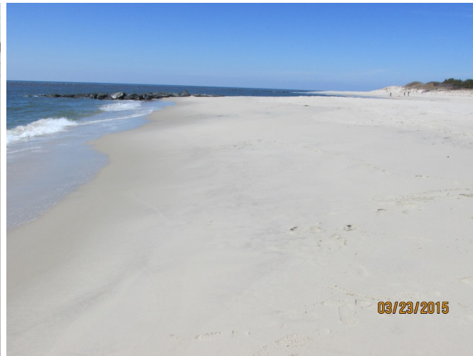
The 2015 photo taken on March 23 shows that the berm appears to have lost a modest amount of width and height. The adjacent groin appears to have less beach around it in 2015.
