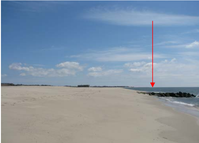
Figure 3. April 2011 shows a wide beach from the bunker to the first groin. Note that with the exception of the seaward end, the groin is buried by sand.
