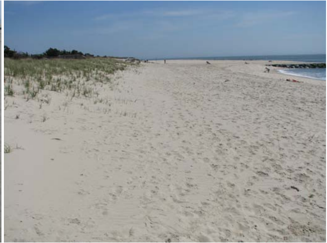
The April 2012 photo shows the accumulation of sand on the northeast (updrift) side of the groin at Coral Avenue.
