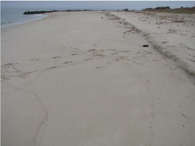
Figure 17. April 2011 the beach has extended seaward to near the tip of the Alexander groin. The beach is now wide enough to support both dune growth and recreational users.
