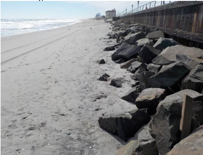
Figure 3a taken October 12, 2016 looking south along the revetment and bulkhead. The beach slopes seaward from the rocks allowing most high tide wave to reach the rocks.
