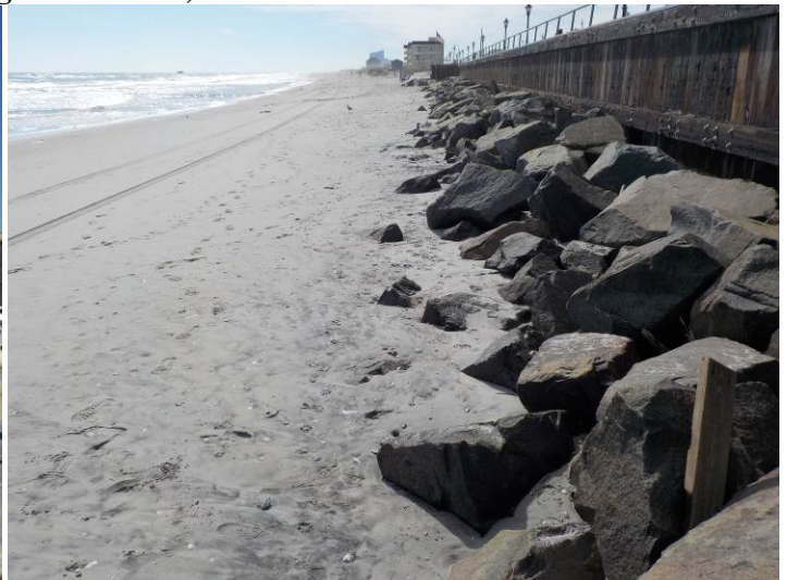
Figure 3b photo above was taken October 12, 2016 showing the significant loss over the past year. Rocks exposed and a hundred-foot narrower beach is present with a generous deposit seen offshore where waves are breaking.
