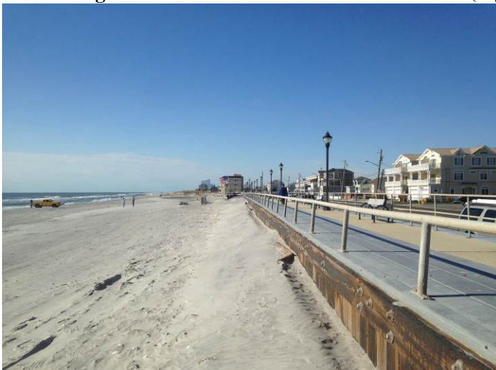
Figure 3a taken October 16, 2015 from the top of the sand against the revetment wall. The wide beach berm still present in spring 2015 has been flattened by storm wave run-up that nearly reached the revetment two weeks prior during the early October northeaster.
