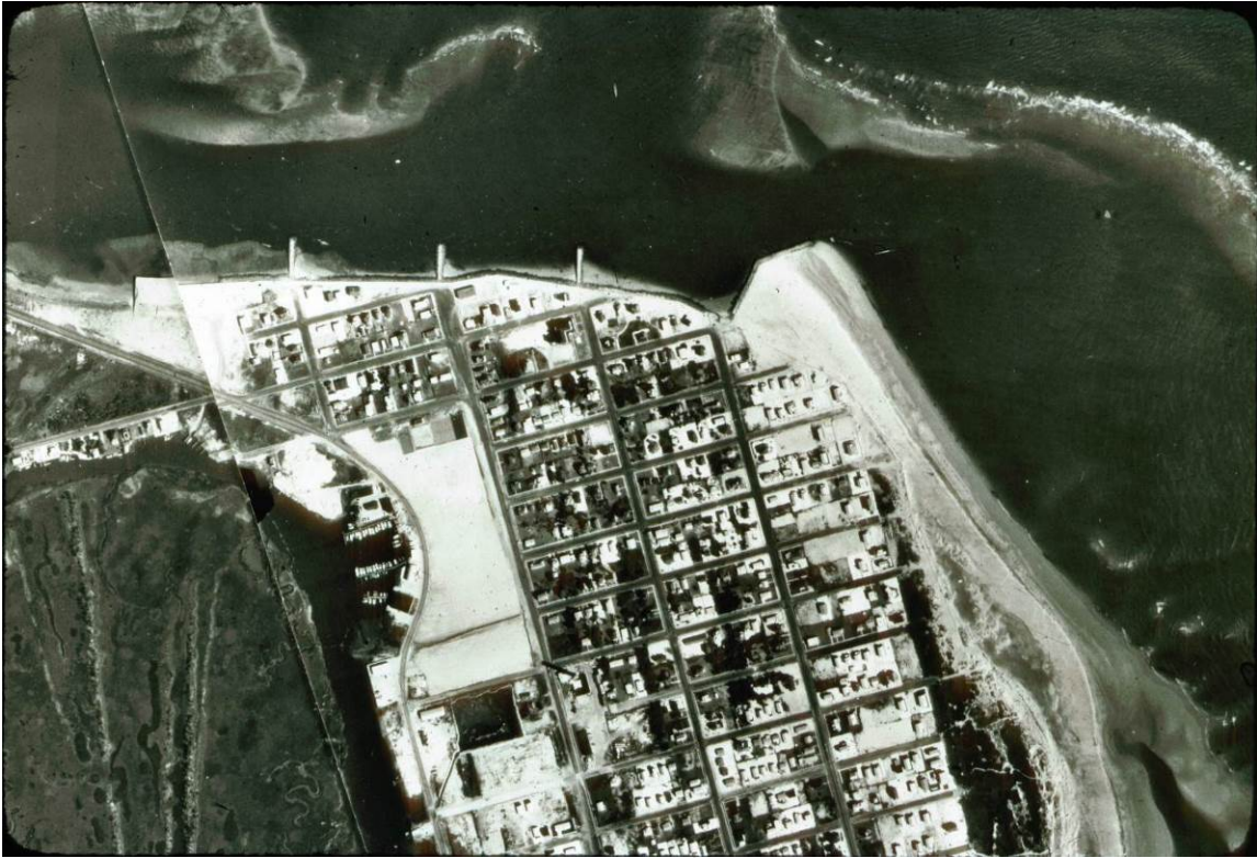
Figure 13. 1971 aerial photograph of Townsend's Inlet after construction of the 8 th Ave. jetty, the rock revetment and 3 short finger groins in the inlet. The main channel lies next to the revetment with vast shoals exposed at low tide immediately northeast of the channel. Note that the seaward parts of the shoal wrap around the inlet mouth and contributed large slugs of sand to the beach lying between the jetty and 17 th Street in Avalon. At this time there was a 465-foot wide vegetated dune system seaward of the end of 17 th Street before reaching the dry, high tide beach. Flood tidal currents and storm wave action moved sand over the jetty into the inlet where the ebb-tidal currents carried it back out to the shoals for eventual return to the north end beach. A stable cycle of sediment was in place. The jetty was also lower in elevation and shorter so that sand did move back into the inlet from Avalon generating a feed-back loop process. Deposits of sand washed over the jetty or around it were rapidly re-positioned by the ebb-tidal currents to the offshore bar and eventually back onto the Avalon ocean beach.
