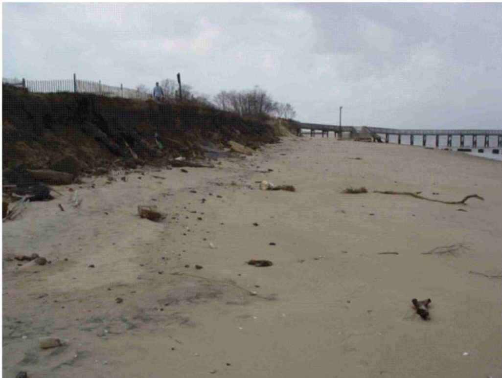
Photoplate 1b. By November 29, 2005 there had been substantial damage done by a pair of northeast storms in mid-October. Erosion destroyed the vegetation and exposed waste rubble used as dune core when the park was upgraded. The beach remained at nearly the same width.
