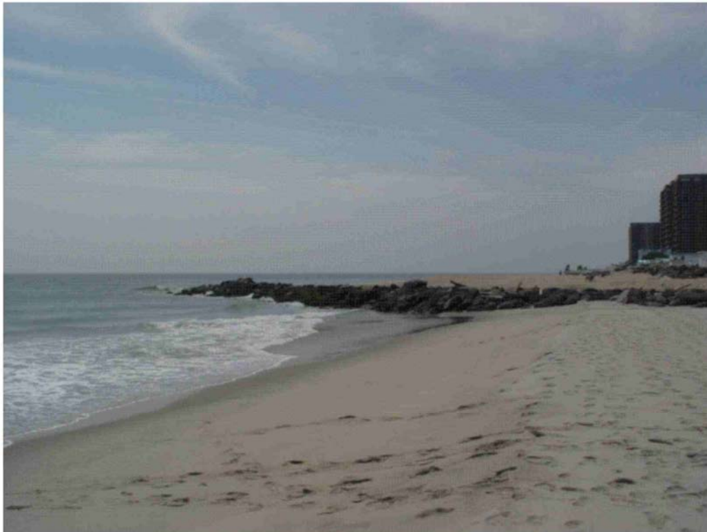
Photoplate 2b. By June 14, 2005 shoreline retreat had exposed the groin again and forced the high tide line back to the rocks south of the groin. The beach continued to erode so that by the summer's end there was a scarp cut into the toe of the dunes north of the groin and well landward of this photograph.
