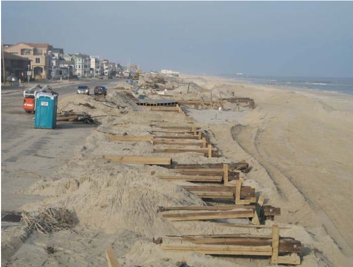
The southern Belmar shoreline was completely overrun by the force of Hurricane Sandy. The Lake Como segment was closed to traffic because multiple pumping pipelines were in place moving lake water back to the sea. Nothing but the supports remained from the boardwalk (left photo, November 12, 2012). 11.23 yds 3 /ft. recovered on the beach naturally by 9/27/2013.
