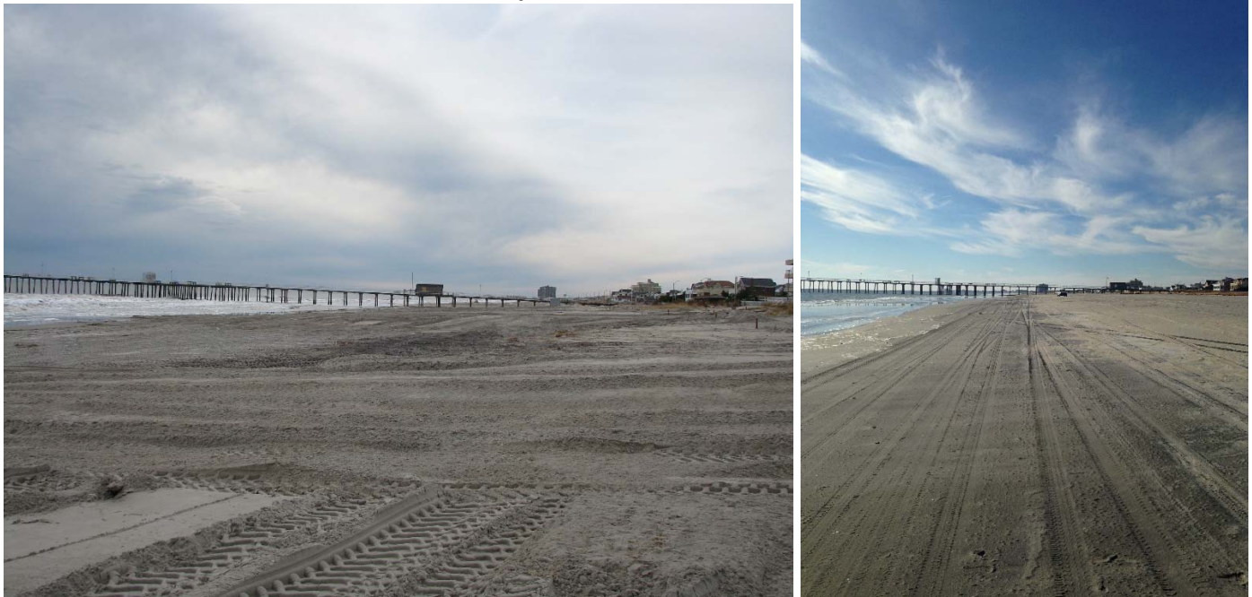
Dorset Avenue site was only minimally impacted by H. Sandy. The losses were within the range of all seasonal changes (left-December 5, 2012). The photo on the right (November 25, 2013) shows the conditions following the Federal emergency fill
