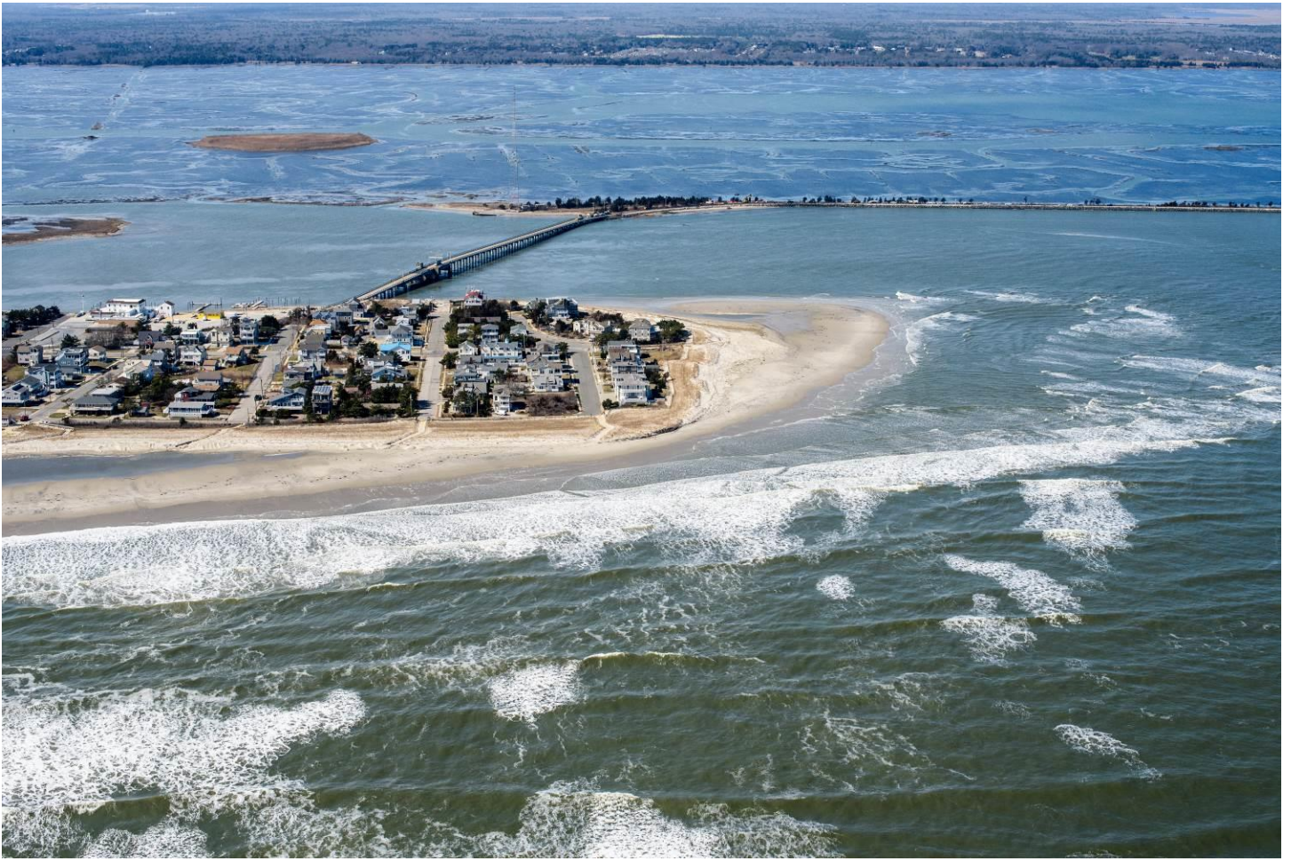
Figure 14. View March 6, 2018 as the second of four northeast storms to impact the NJ coast was getting underway during a spring tide. Note the flooded salt marshes in the bay. The very northeastern corner of the dunes at Seaview Avenue have been scaped, but offshore bar sand added to the beach in December is still present (photo by Ted Kingston).
