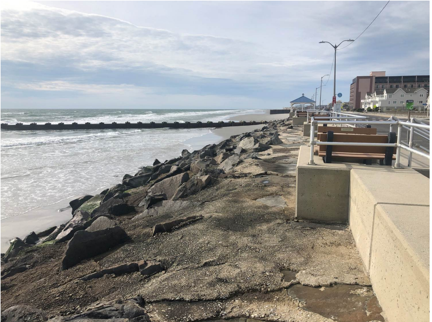
Figure 6. View to the south taken November 7, 2019 showing that the waves at low tide still reach the revetment. The slope offshore is relatively gentle, but not suitable for recreational use.
