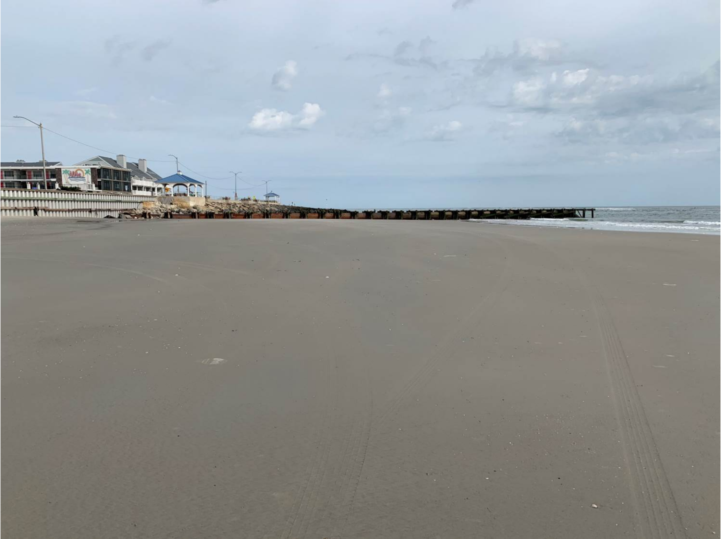
Figure 8. The view toward the jetty from the lower beach near low tide shows that there is no dry beach as of October 2019.
