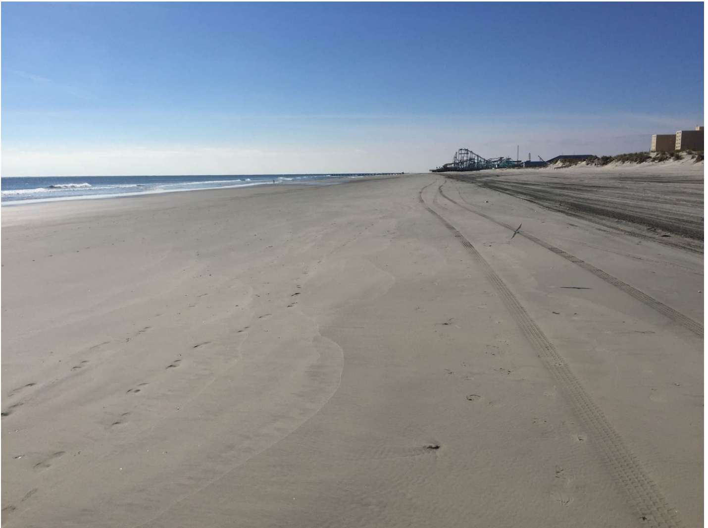
Figure 16. View to the south along the upper beach on October 25, 2019. Beach flattening has moved the wet/dry surf line close to the dunes. While no erosion of the dunes has occurred yet, the narrow beach where the most visitors tend to gather presents a space problem for the coming season.
